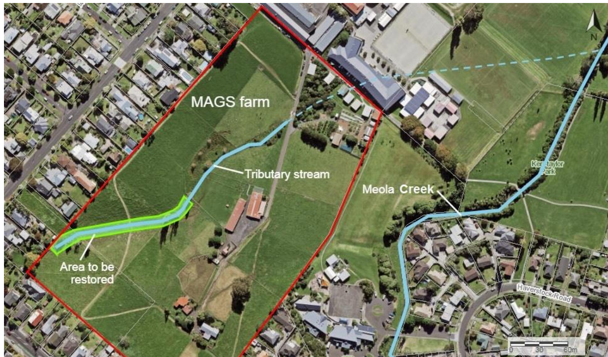
Figure 3 Indicative MAGS farm restoration area (~1,770m 2 ), as proposed under the Waititiko – Meola Creek Enhancement Plan
