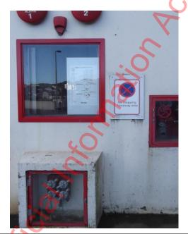
Building riser inlets at bottom of photo  $\rightarrow$ Photo - NZFS
