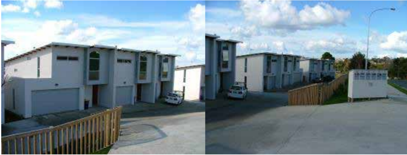
Figure D-22: Slip lanes at the front of a site and at a lower level to the road create a hostile pedestrian environment
