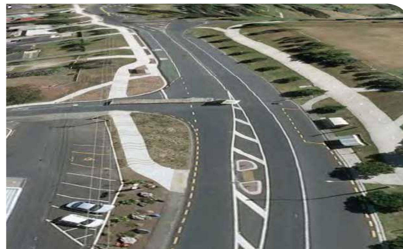
Figure 7-4: Northbound Approach to Forrest Hill Road roundabout
