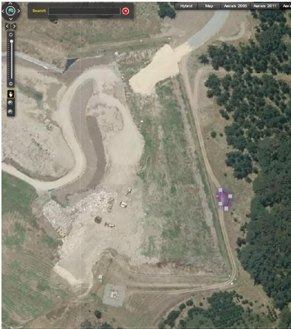
Figure 1 – Approximate location of leachate breakout on 12 May 2017.
