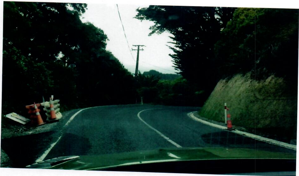
Photograph 1: Power Pole at ch. 660
