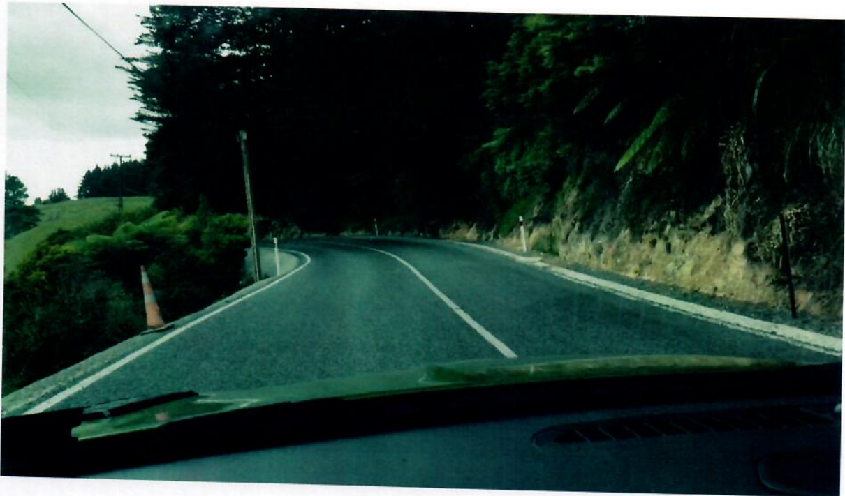
Photograph 8: Steep Fall on Northern Side of Twilight Road
