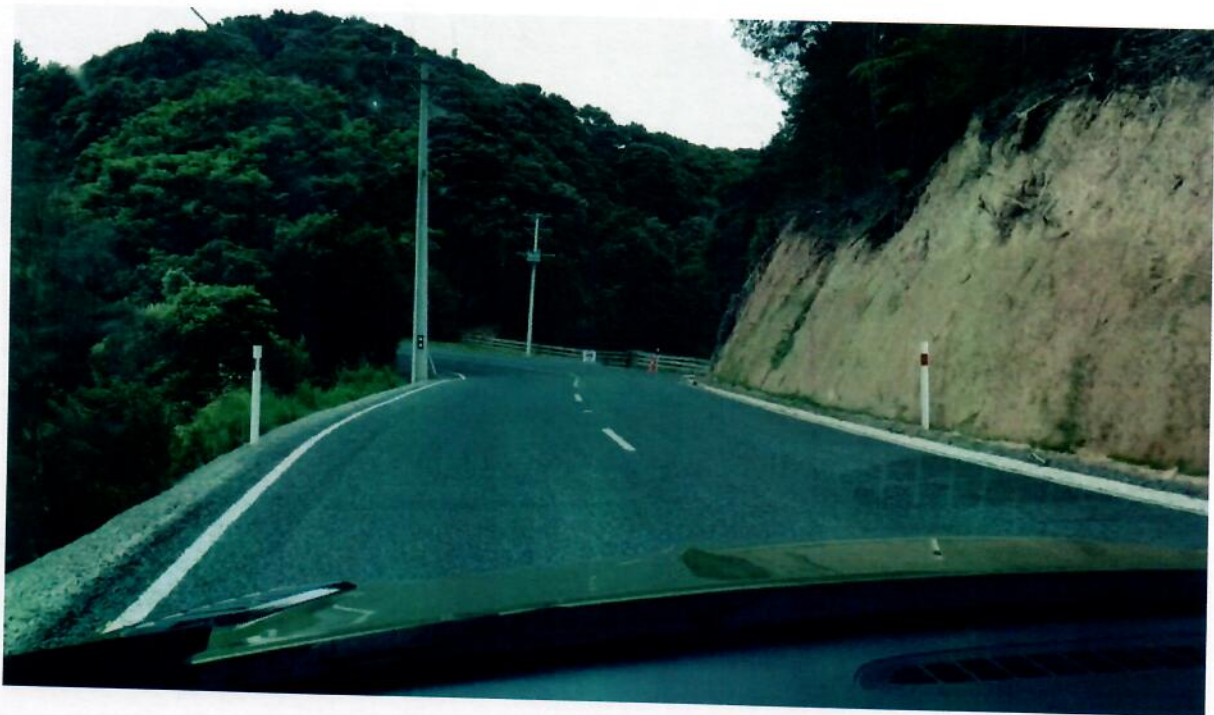
Photograph 6: Power Pole at ch. 1160
