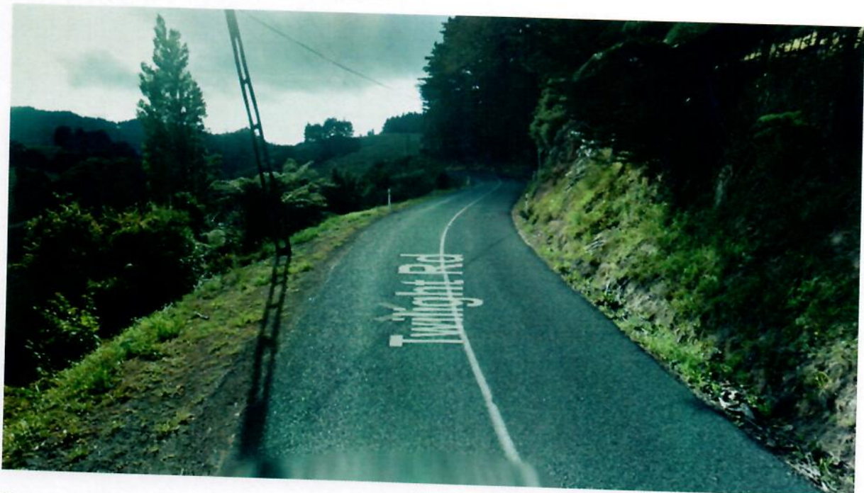
Photograph 7: Power Pole at ch. 760 (prior to widening)
