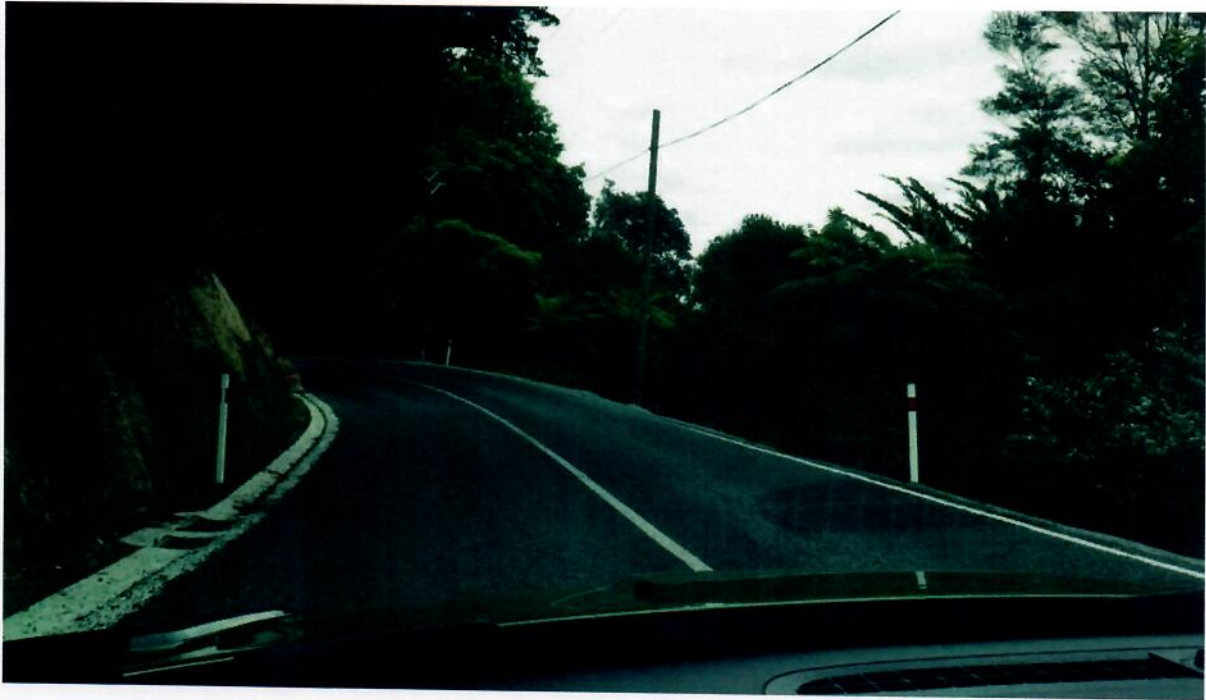
Photograph 9: Tree on Inside of Bend at ch. 650
