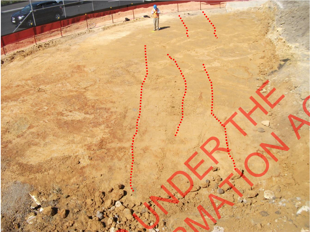
Photograph 6 & 7: Indicative spacing and distribution of large cracks (1.5-2m)
