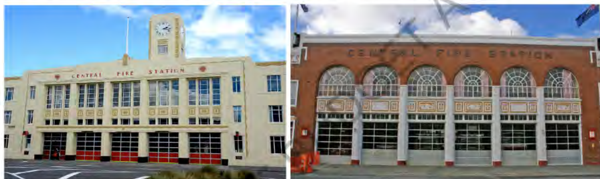
Figure 7 Images of Wellington and Dunedin Fire Stations
