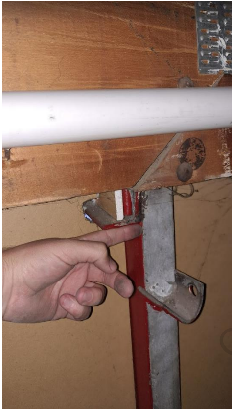
Bottom flange of appliance bay rafter connected to steel post.
