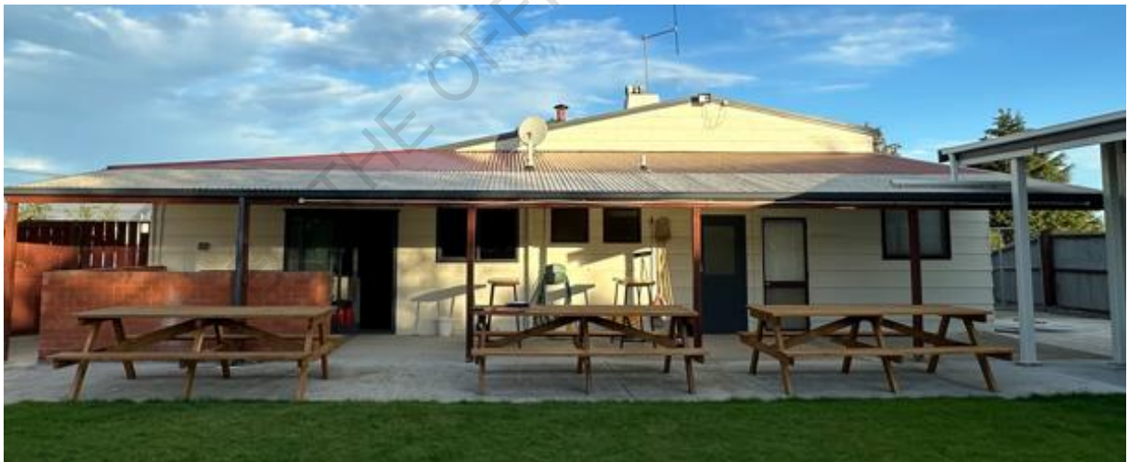
Exterior weatherboard and corrugated steel cladding.
