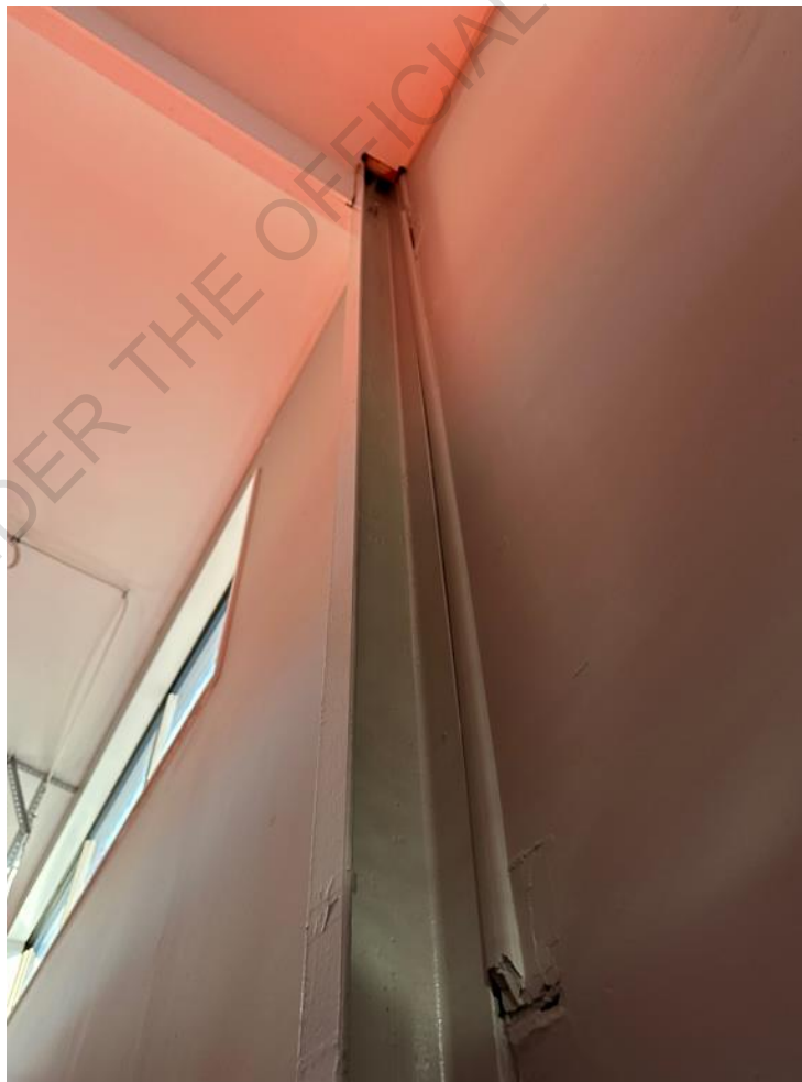
Appliance bay steel portal frame.
