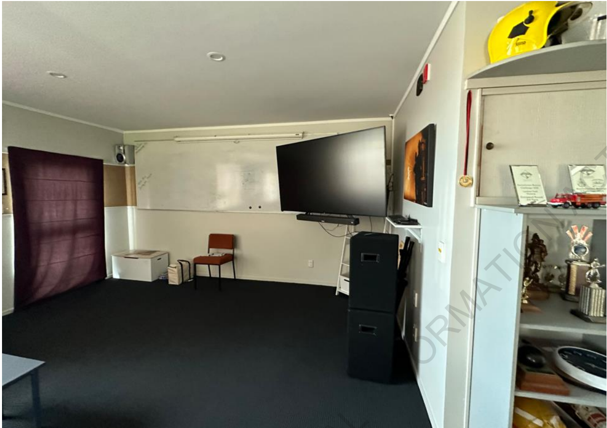
Plasterboard lined timber-frame walls.
