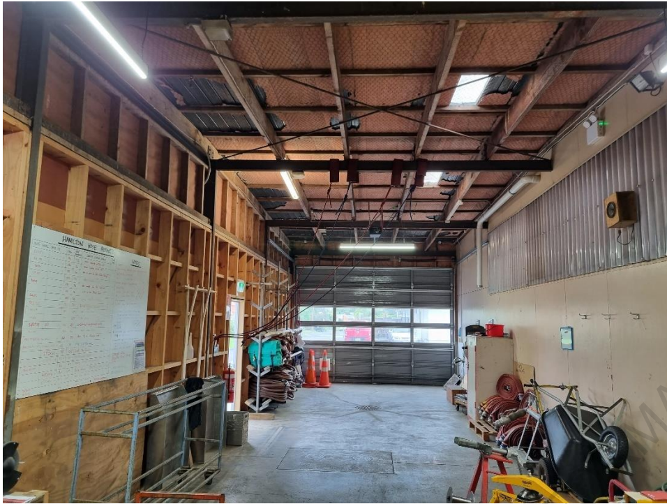
Photo 5 – Internal view of Appliance Bay 02
