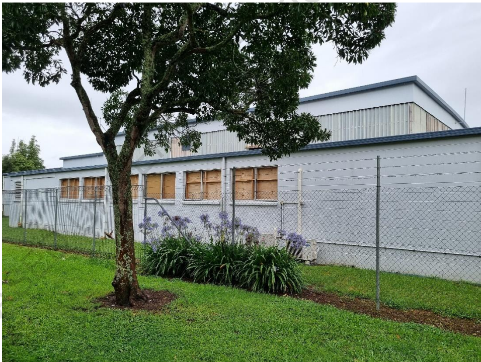
Photo 2 – Rear (south) elevation
