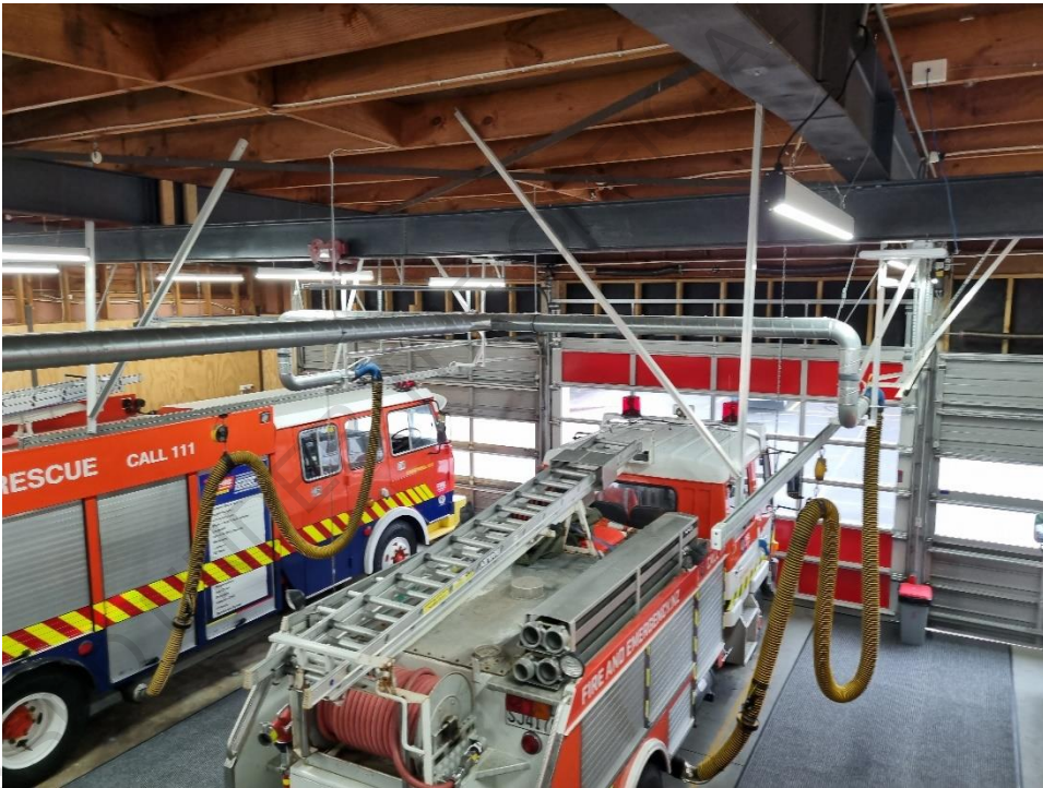
Photo 4 – Internal view of Appliance Bay 01
