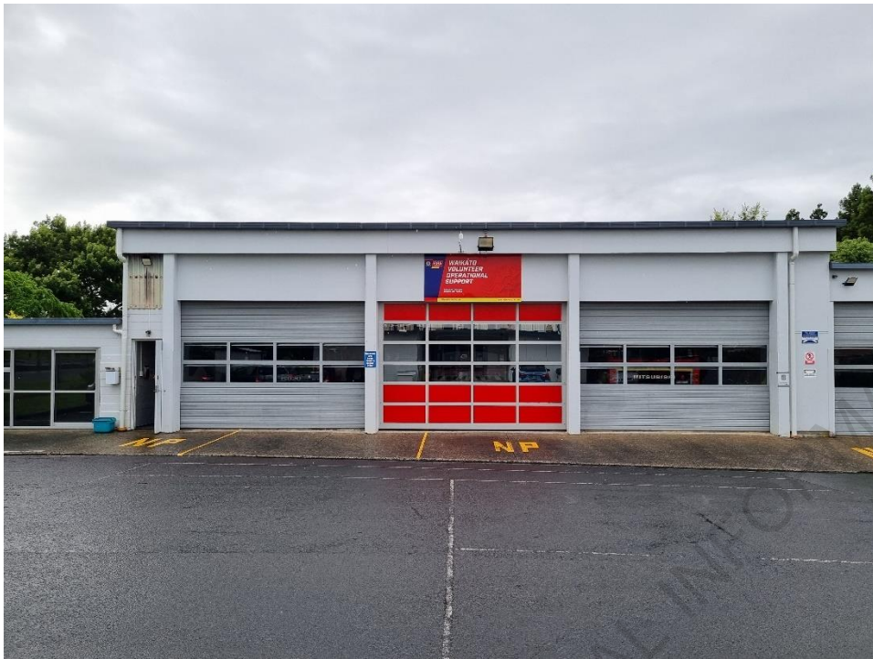
Photo 1 – Front (north) elevation of the Operational Support Building
