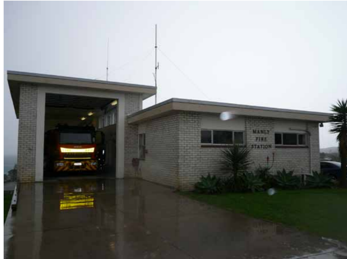
Whangaporoa Road, Manly
