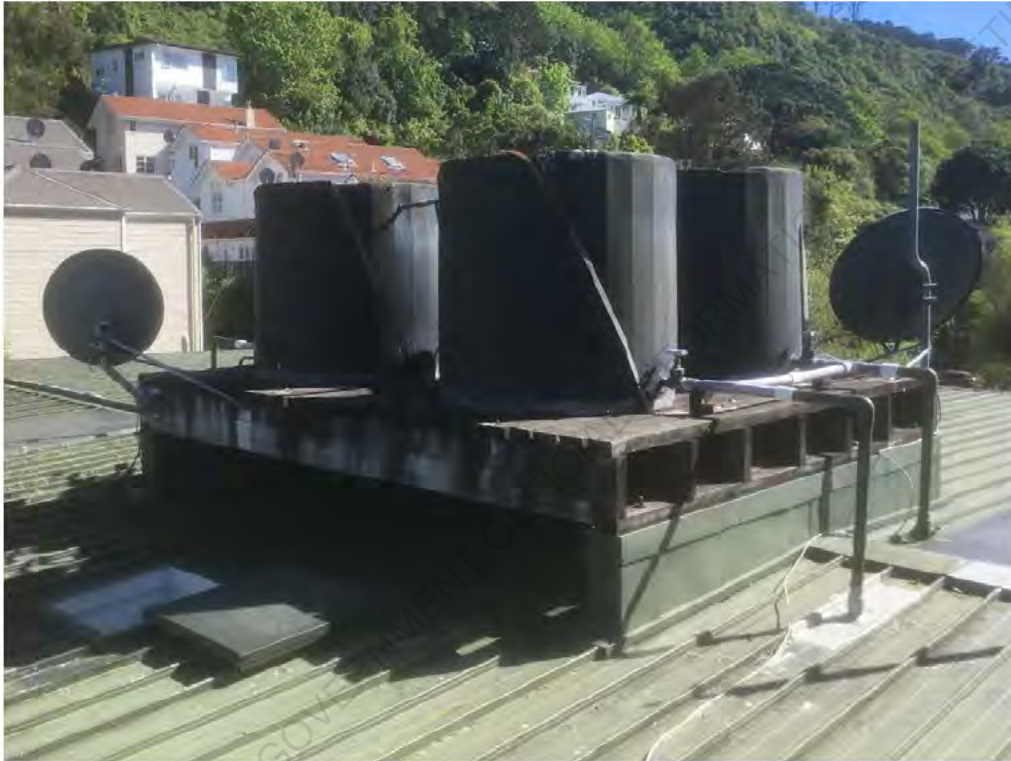
Figure 13: Roof tank support structure
