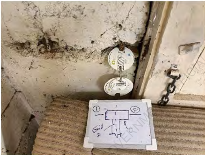
Condition of the garage wall piers
