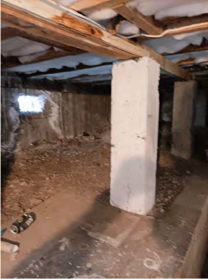
Typical interior pile and general view of rear foundation wall
