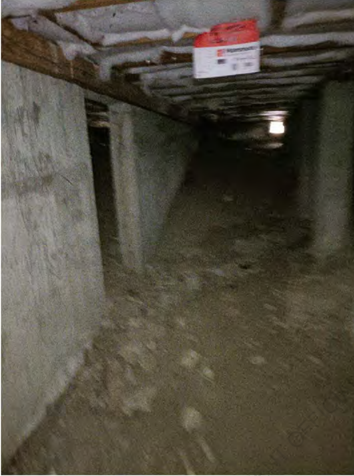
Typical interior concrete foundation wall
