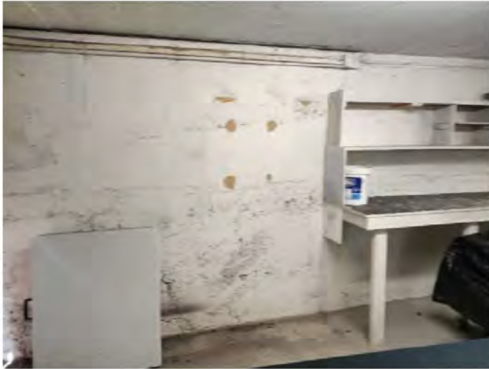
Typical condition of visible interior concrete at garage level.
