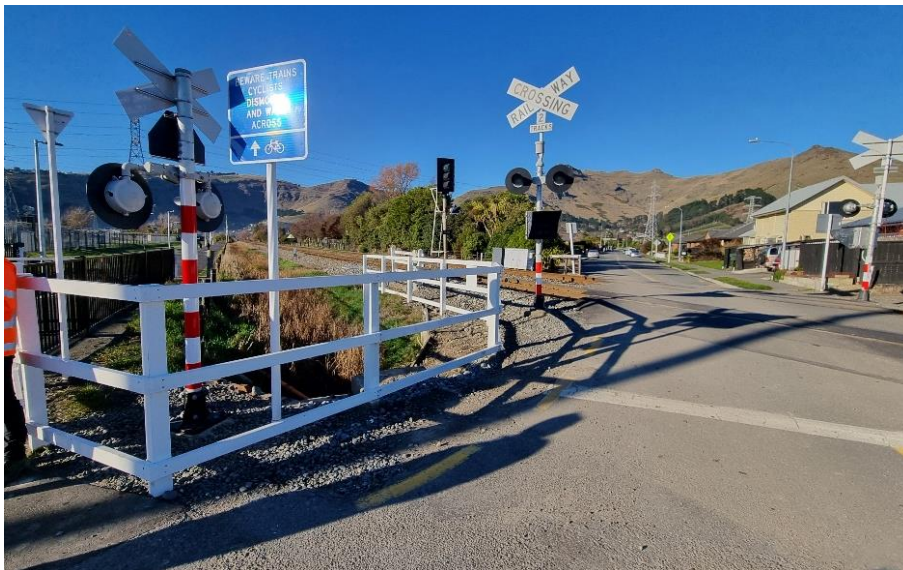
Figure 4-15: Fenced culvert, with set of FLB facing the eastern MCR approach
