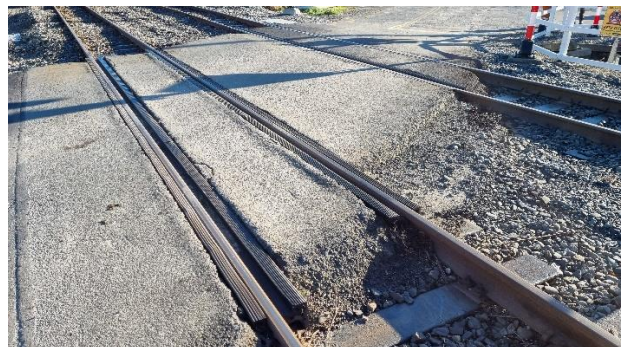
Figure 4-12: Flange gaps, EPflex on track panel
