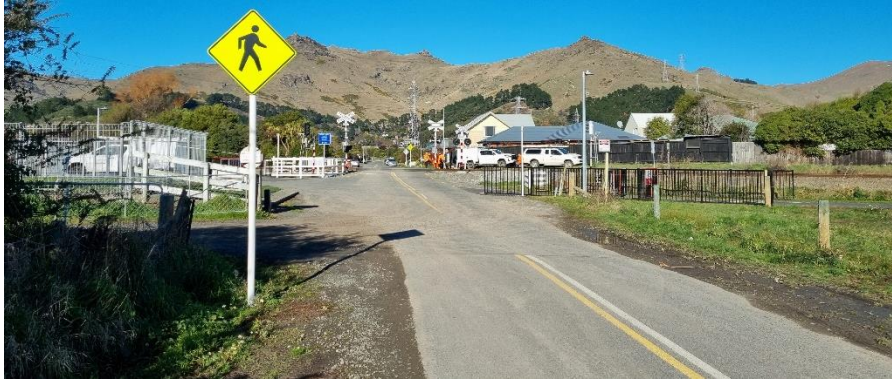
Figure 4-17: Pedestrian warning sign (north approach)
