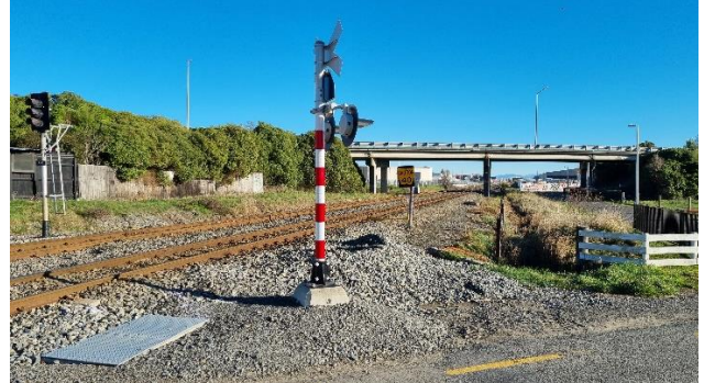
Figure 4-8: FLB with "RAILWAY" crossbuck sign and west track sightline on the northern approach
