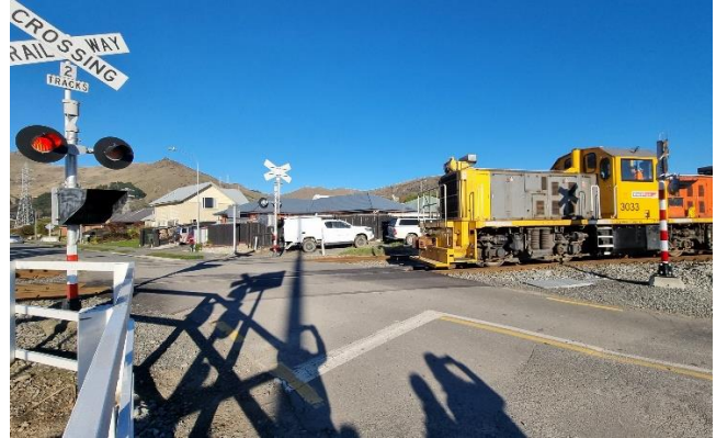
Figure 4-4: Northern approach to level crossing from northeast angle
