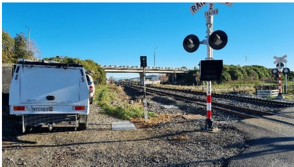
Figure 4-5: FLB with 'RAILWAY' crossbuck sign and West track sightline on the southern approach
