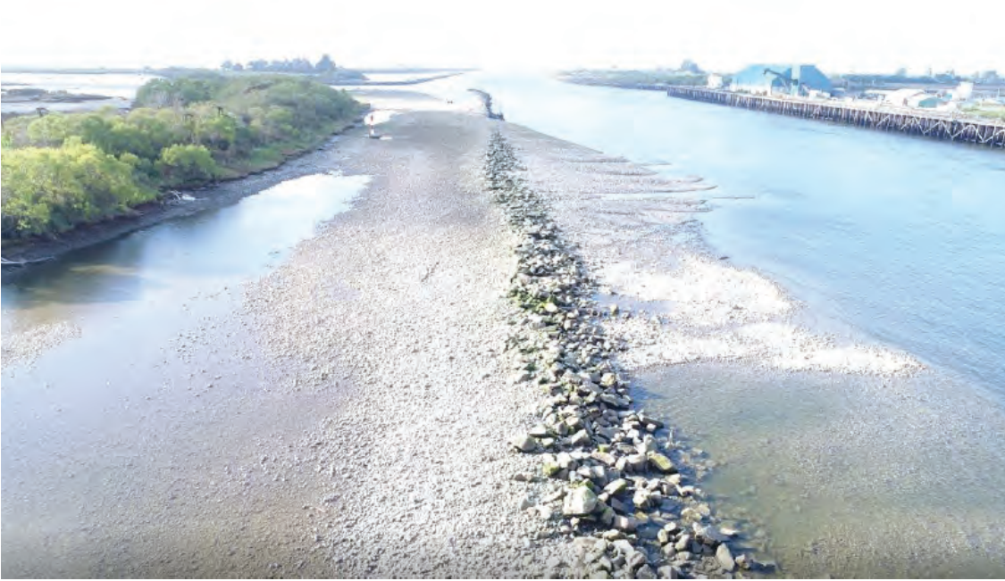
Figure 4-2: Gravel Build-up at Half Tide Wall
