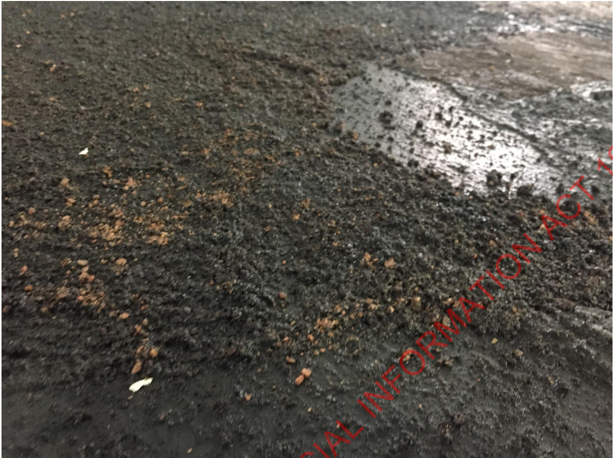
Image 5 - abrasive grit material designed to increase friction of the surface and give cattle more grip, but resulted in lameness
