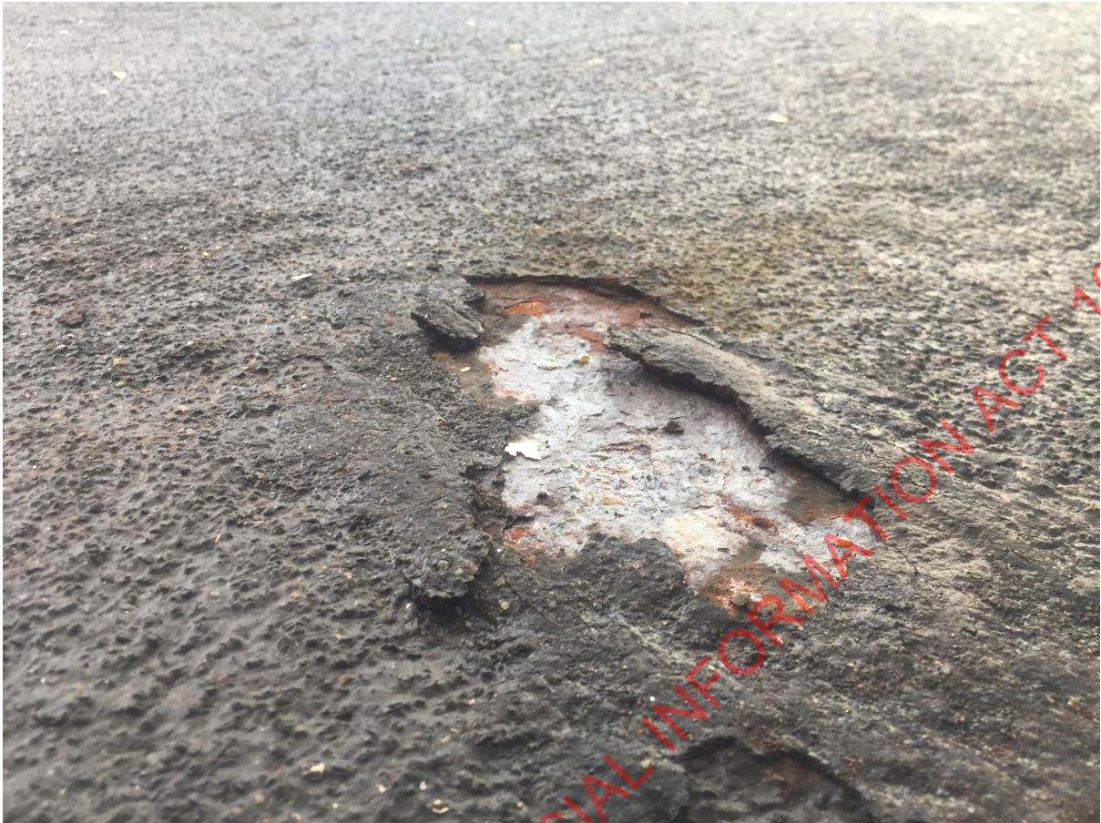
Image 4 - damage to pen flooring only evident after ship had been cleared of cattle and effluent
