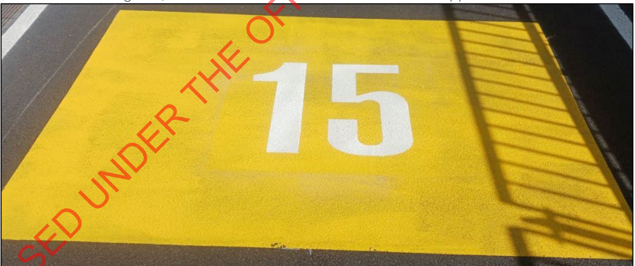
Figure 41: Advisory speed marking on approach to Petone Station.
