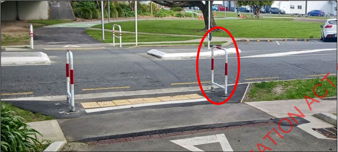
Figure 22: Pharazyn Street shared path crossing with right-hand hold rail on western side circled.
