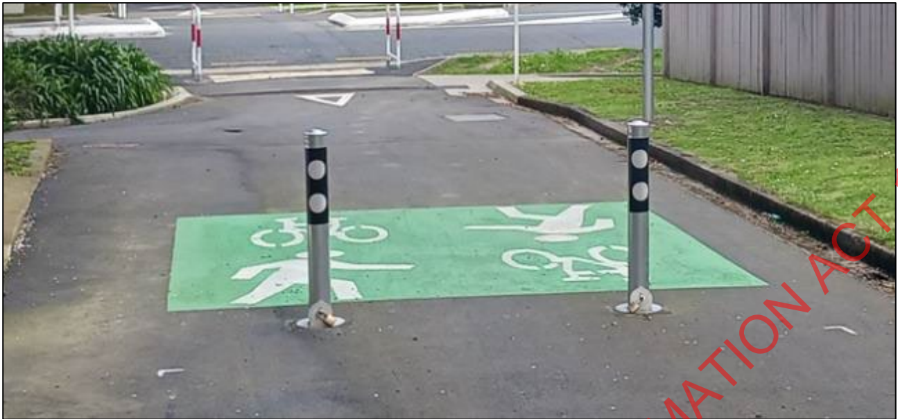
Figure 23: Bollards on shared path west of Pharazyn Street.
