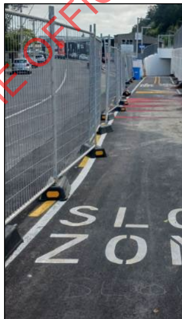
Figure 21: No permanent physical separation between cycle path and traffic lane.
