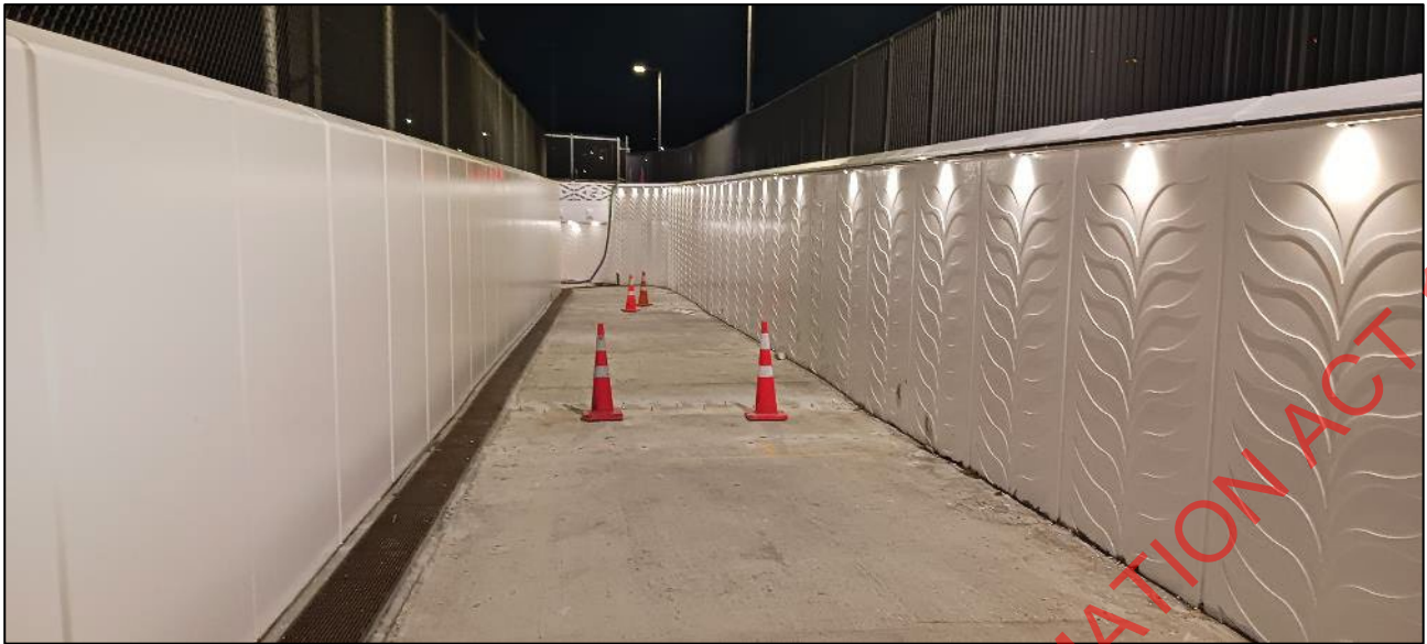
Figure 25: Entrance to Petone underpass at either end.
