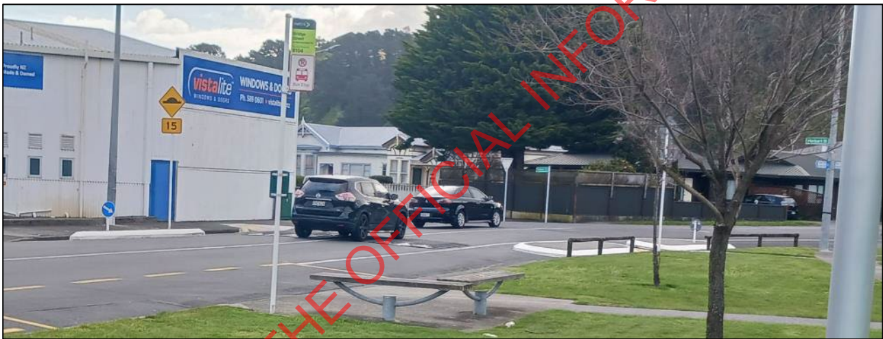
Figure 17: Speed cushions near Bridge Street crossing with vehicles driving along centre line to avoid.
