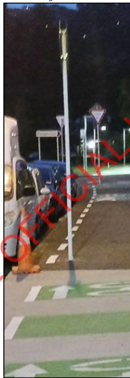
Figure 20: Example of WU61 sign pole located within shared path.
