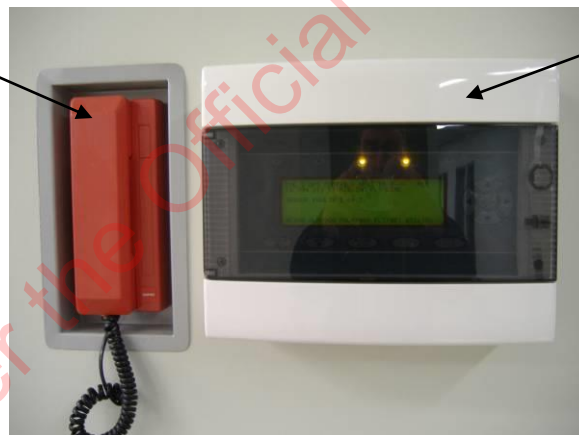
Mimic panels installed in Wellington Regional Hospital
