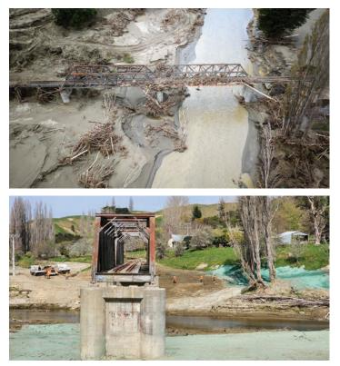
South of Waikou a large body of water built up behind the rail embankment during the cyclone, then broke through it shortly afterwards before we could get any machinery to the site. The pictures below show the scale of the original water build up and the mitigation work that followed. exposed material from further weather damage. Damaged bridge piers and spans have been removed as they were unstable and damaged track was cut away.
