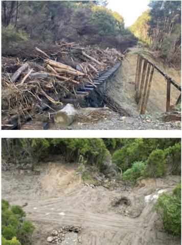
Before and after pictures of a major culvert and embankment washout north of Tutira. This massive, 20-metre-deep washout left around 60 metres of unsupported, hanging track. Works have since been undertaken to remove the track and stabilise the slopes at either end to prevent further deterioration.
