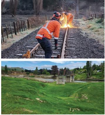
Work ranged from removing hanging track, trimming back unstable washed out embankments, reopening drainage paths to manage water flows and creating access tracks for plant to get through the site.
