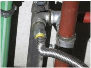
9. Terrace Building, Level 7: The understairs sprinkler head is plugged off.
