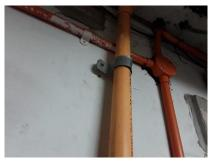
6. Level 1, kitchen serving area: Sprinkler head dropped from ceiling and ceiling tile lifted. Contractor to confirm adequate pipework support. Refer photo below.
