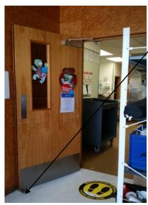
During the inspection the fire door from the kitchen that leads to the service stairwell was found wedged open. This was noted in the 2020 / 2021 report. This door is required to stay closed at all times.
