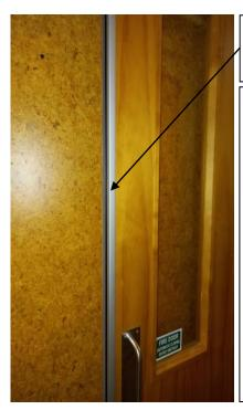
Existing fire / smoke stop doors with improved smoke stopping seals installed.
