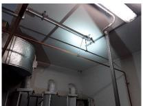
5. Level 16, Plant Room: Pipework support not securely attached to the wall. Refer photo below.
