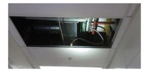
8. Tower Building, Level 7 main kitchen: Flexible dropper visible through the missing ceiling tile above the wash-up bench beside gas grill has too tight bend radiuses. Refer two photos below.
