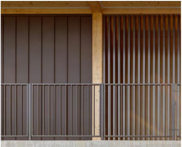
ERIC TWEEDALE STADIUM, NEW SOUTH WALES
