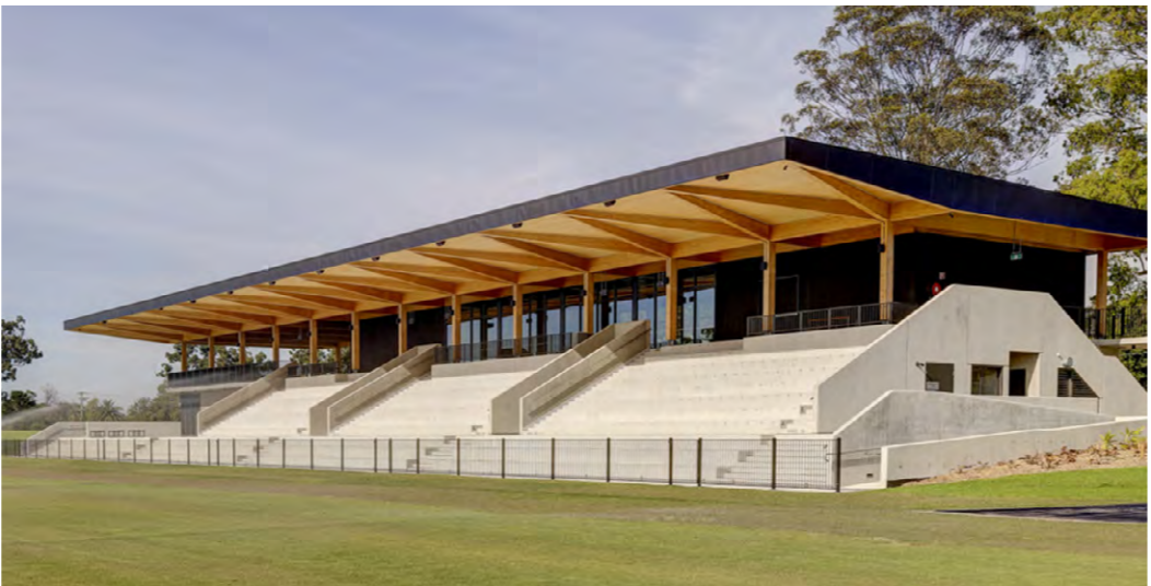
ERIC TWEEDALE STADIUM, NEW SOUTH WALES
