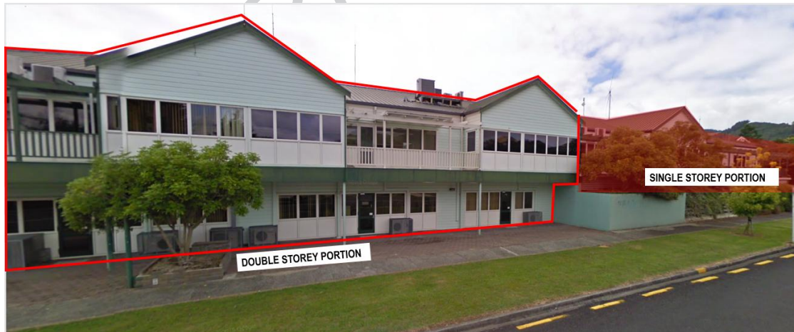
Figure 1: Waitomo District Council Building (Google Maps Image)
