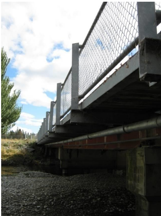
Photograph 7.2.2: SH 8 Twizel River Bridge
