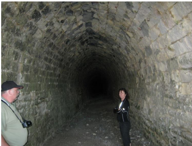
Photograph 7.3.1 Rail tunnels at Tunnel Hill
