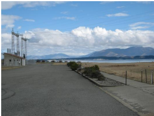
Figure 3 Tekapo B Power Station
