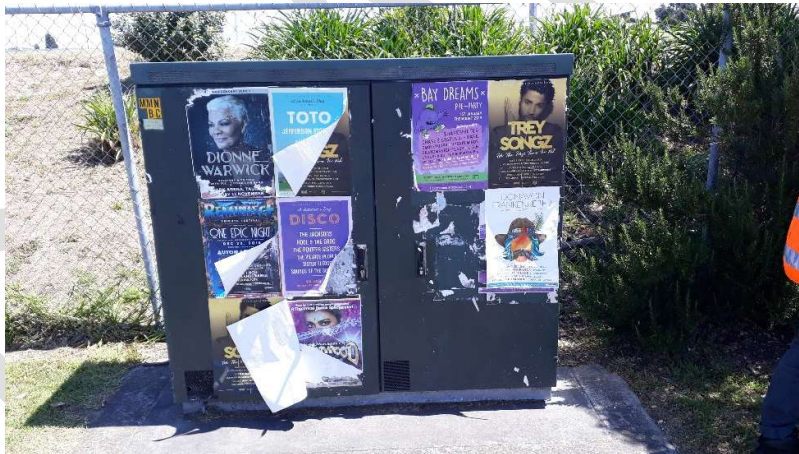
Figure 30: Existing Chorus Box to Remain
