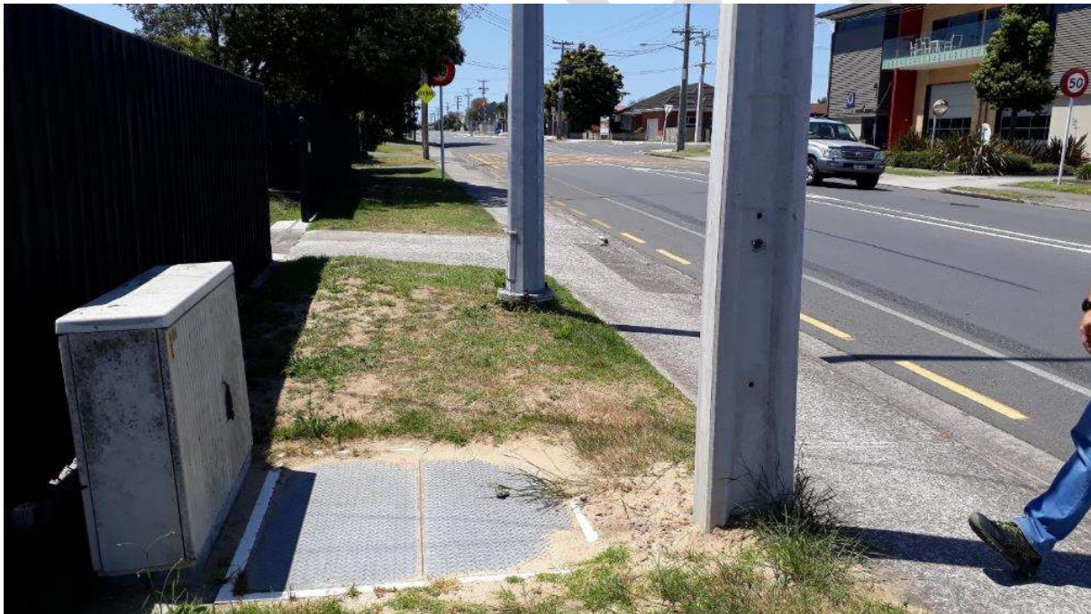
Figure 5: Recently Installed Power Pole
