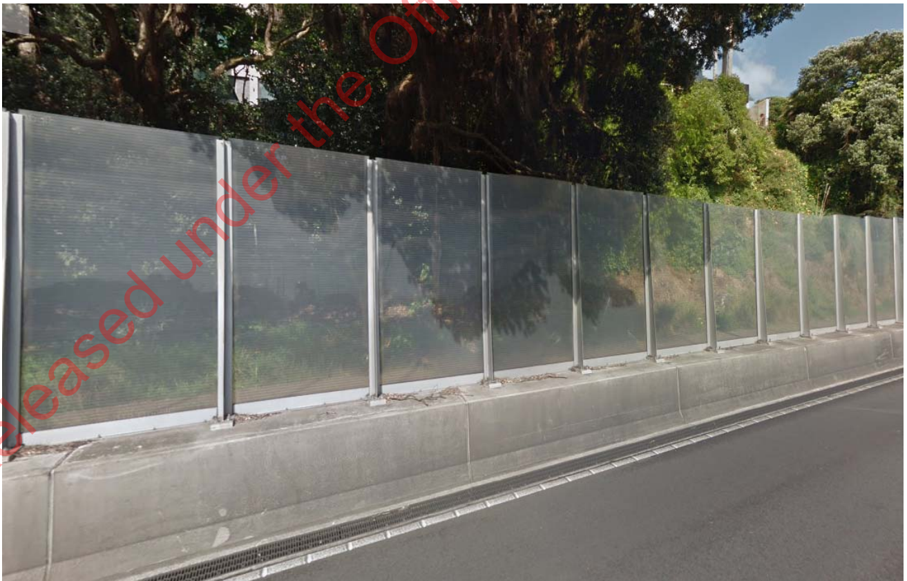
4. Existing barrier to south of Auckland harbour Bridge
