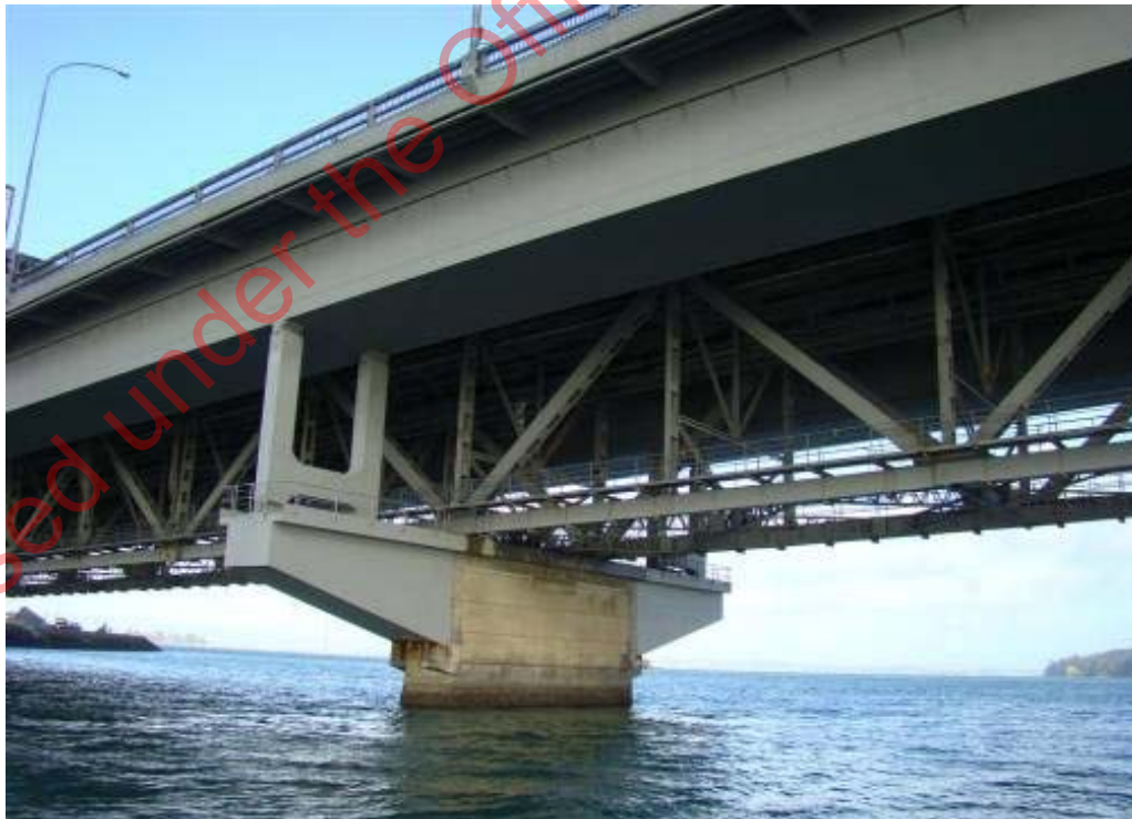
2. View of underside of extension construction
