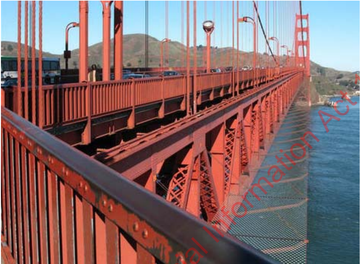
Golden Gate Bridge horizontal barrier system
