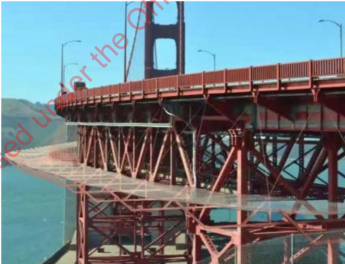
Golden Gate Bridge horizontal barrier system
