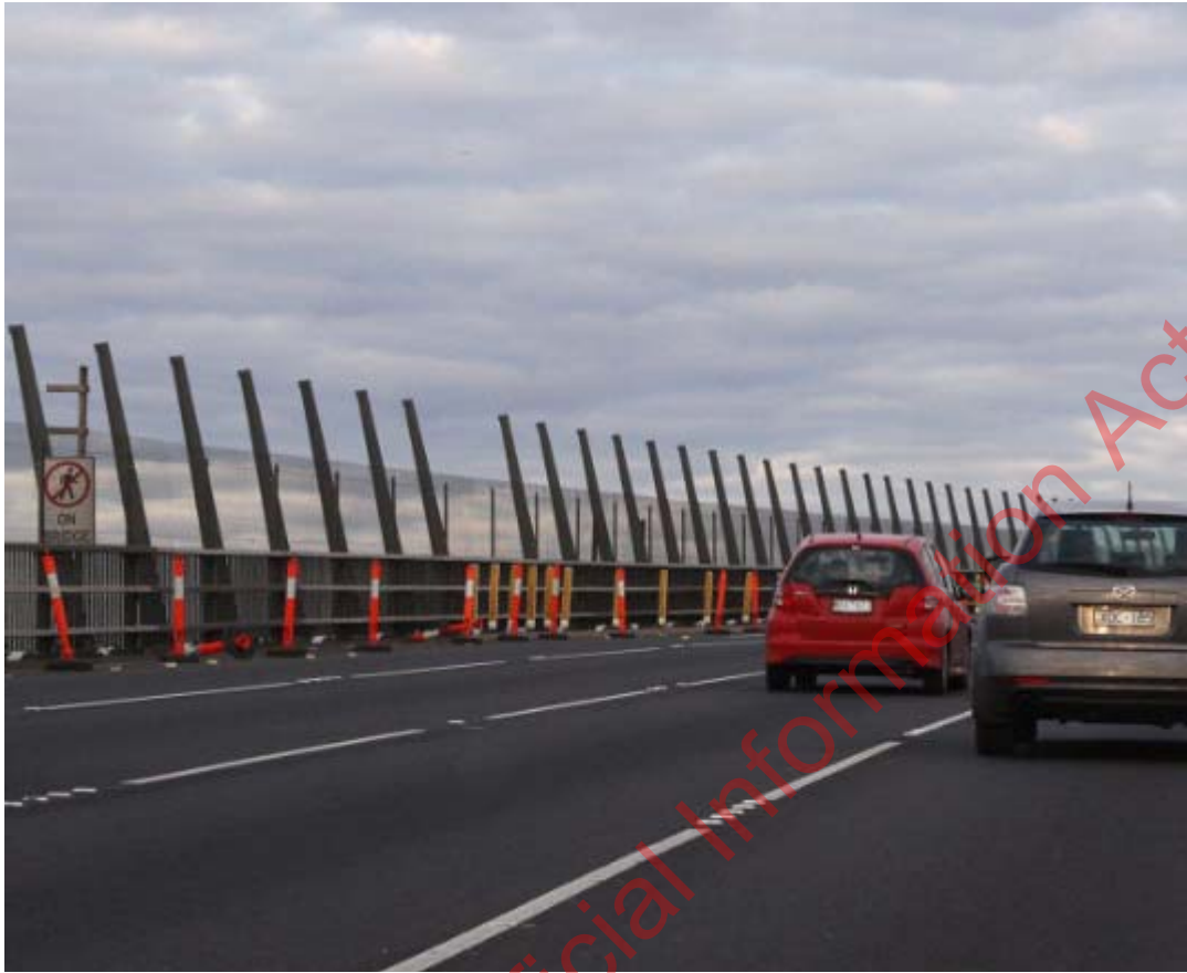
West Gate Bridge outward raking barrier system
