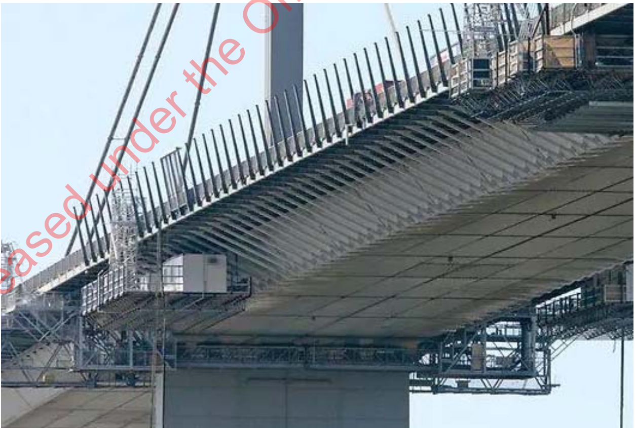
West Gate Bridge outward raking barrier system
