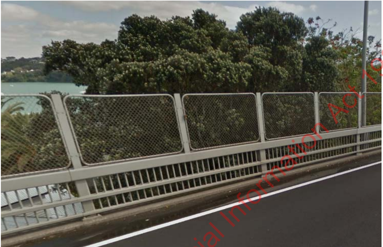
3. Existing low-level barrier along majority of structure
