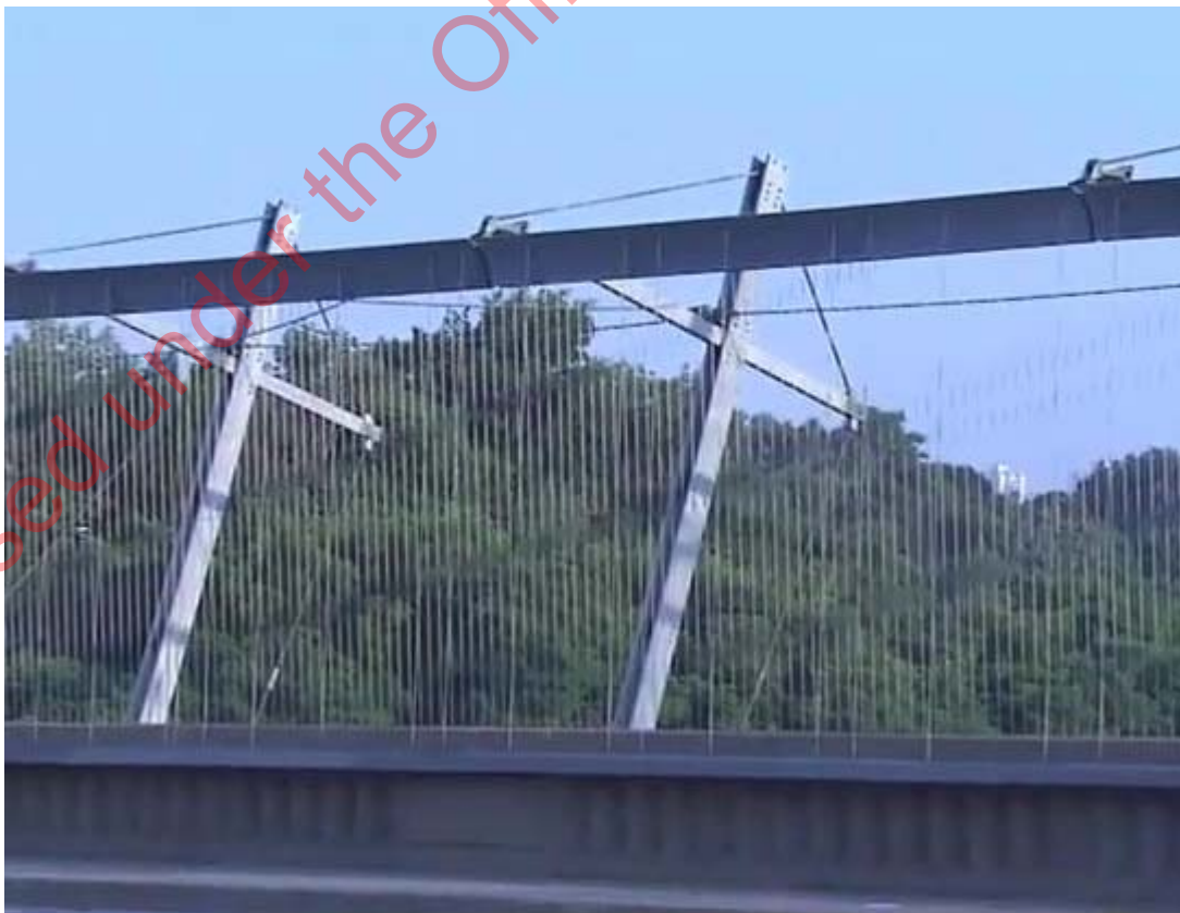
Bloor Viaduct Vertical barrier system
