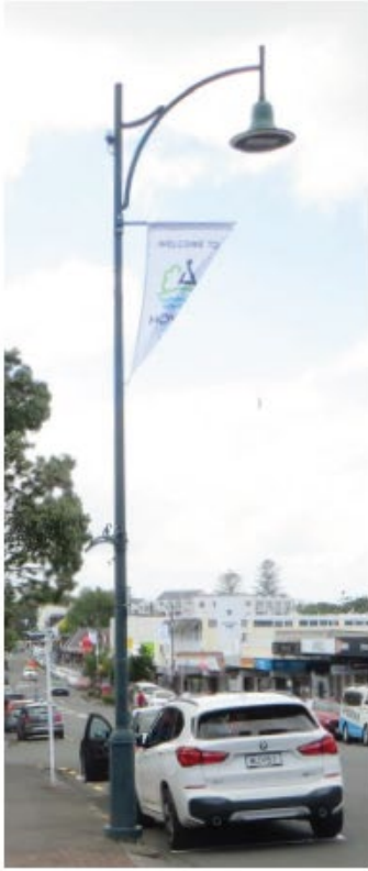
EXISTING STREET LIGHT
