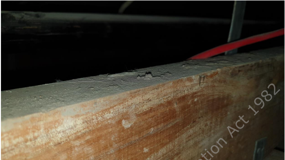
Example of dust in level 10 ceiling.
