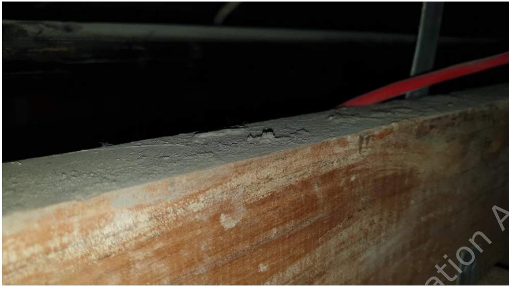
Photo 3: Example of dust loading on surfaces within ceiling space above level 10 lobby to access hatch.
