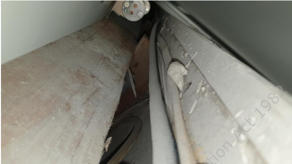
Level 10 through perimeter gap
