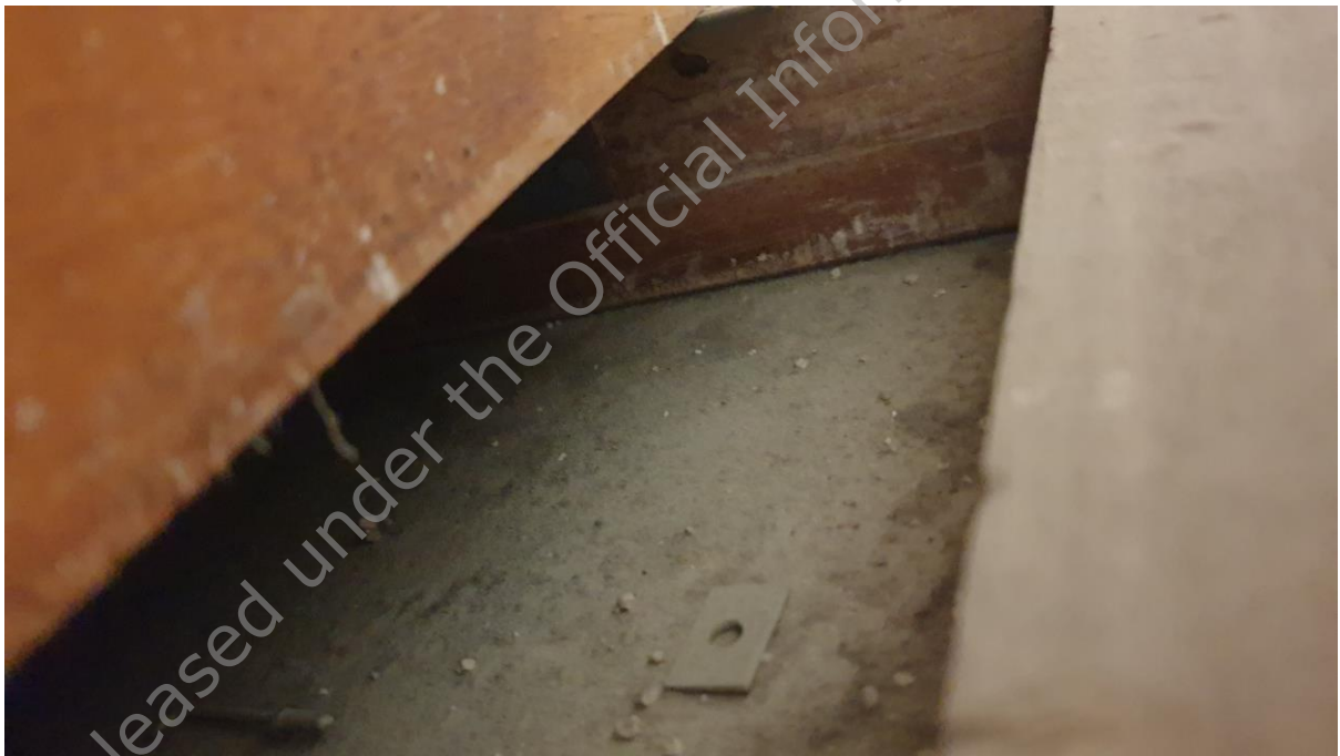
Level 5 through perimeter gap'
