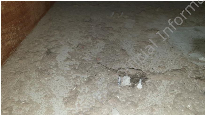
Photo 1: Cement based sheeting above level 10 ceiling.
