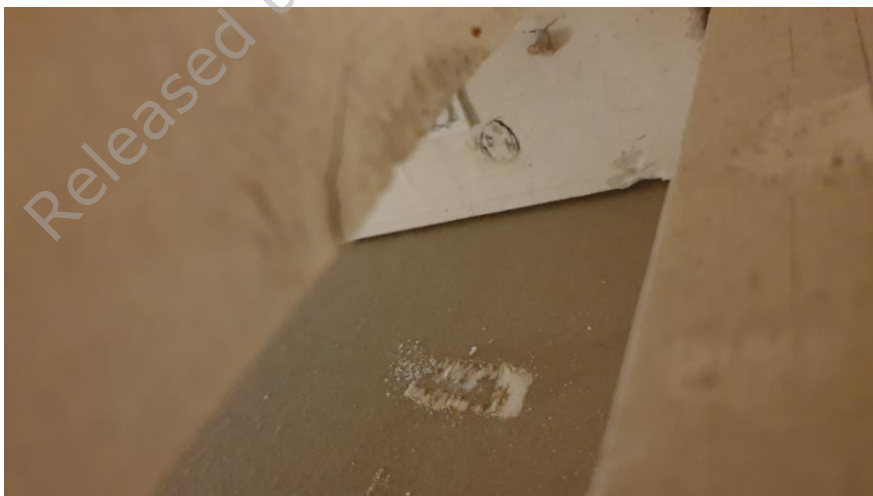
Photo 2: Example of plasterboard ceiling levels 6 – 9.
