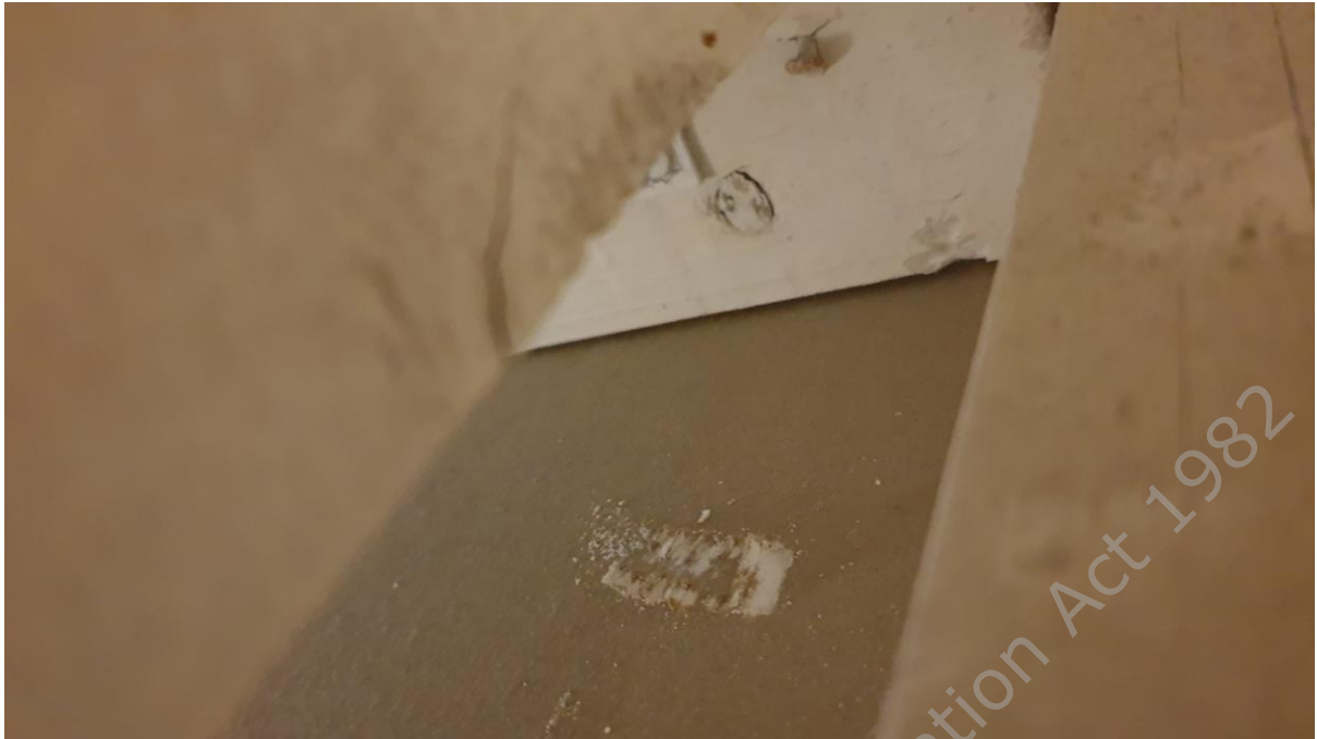
Level 6 through perimeter gap
