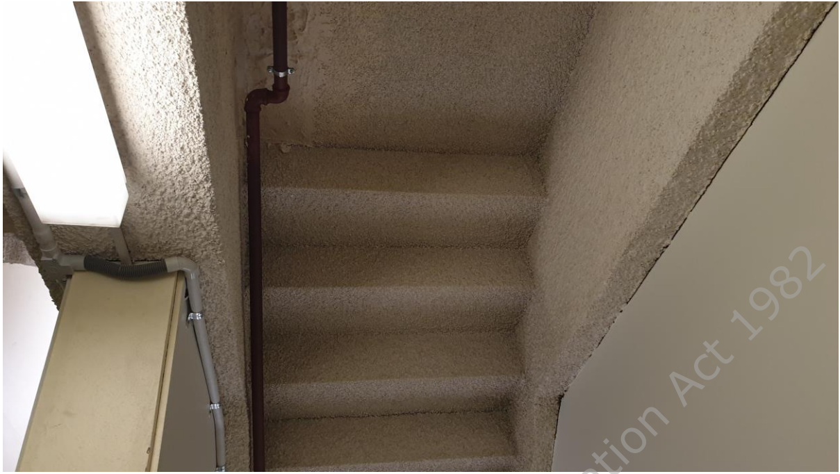
Stairwell spraycoat
