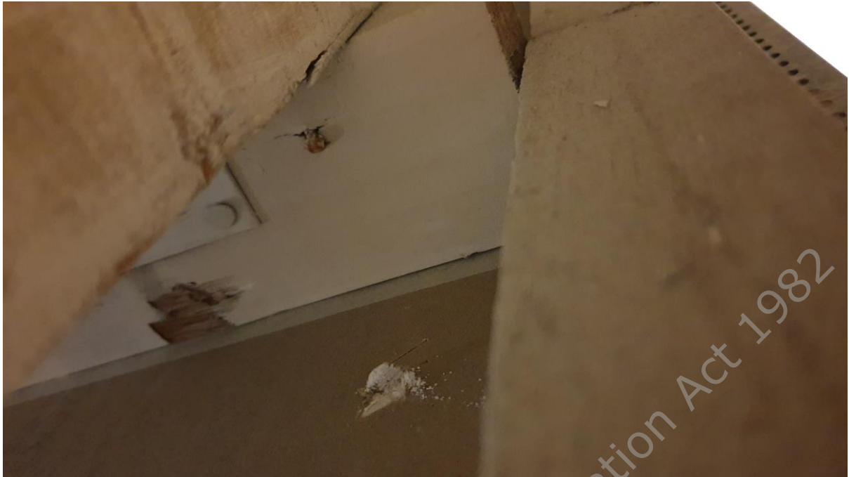
Level 8 through perimeter gap
