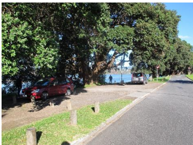
Figure 4-17: Existing car park in poor condition
