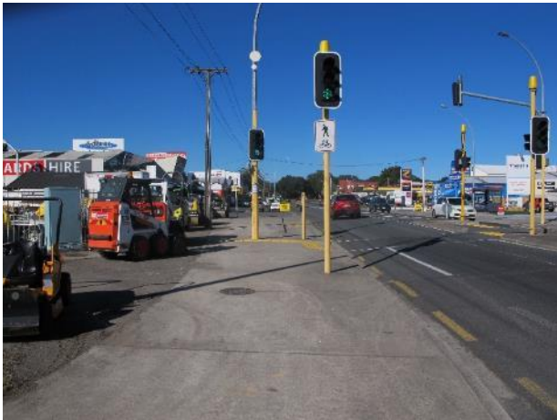
Figure 4-9: Burrows Street Intersection – Kennards Hire. Note large machinery within the road reserve.
