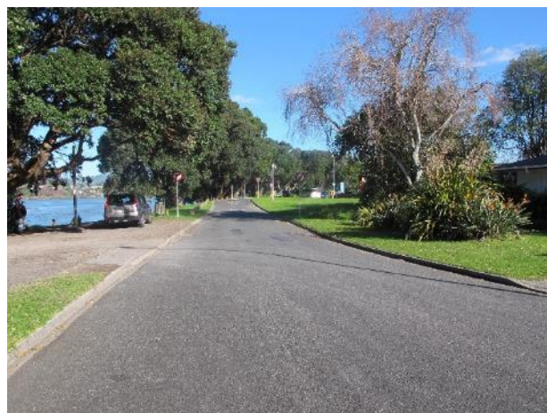
Figure 4-18: Poor access onto Turret Road
