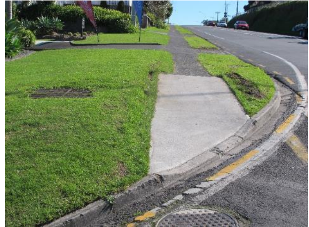
Figure 3-2: Large telco pit at Scantlebury Street intersection that has not been identified for lowering. The designed path will not achieve required gradients for all users.
