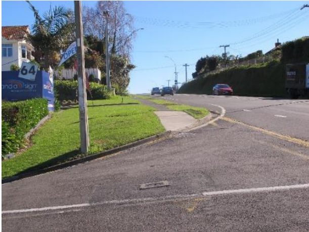
Figure 3-1: Scantlebury Street intersection. Shared path requires flattening to achieve appropriate gradient for mobility impaired users.
