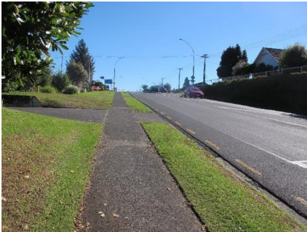
Figure 4-6: Grace Road intersection approach. Note vertical curve to be considered to achieve appropriate gradient for mobility impaired users.
