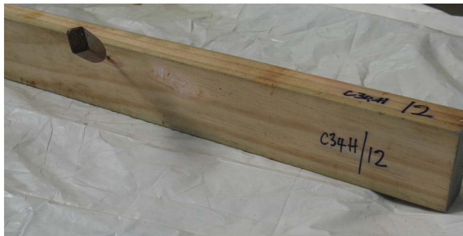
Figure 20 – HMC sample C34H/12 treated with copper naphthenate on four sides after 159 weeks exposure. Decay, probably originating from the pre-treatment decay feeder block has broken through the preservative treated envelope and is beginning to spread along the sample surface.
