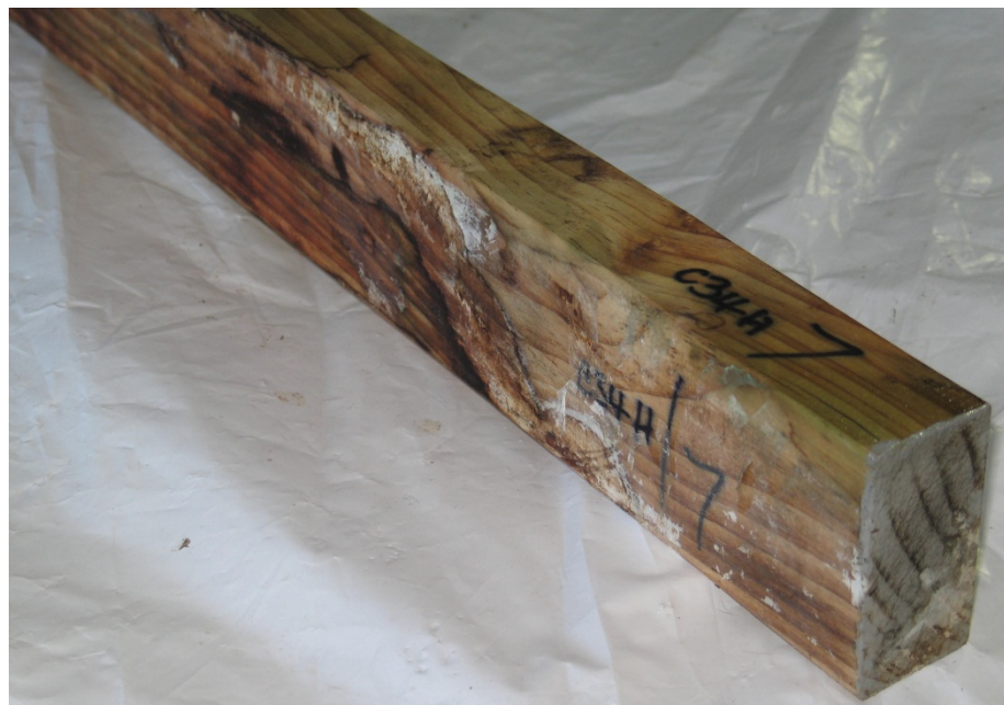
Figure 22 – HMC sample C34H/7 treated with copper naphthenate on four sides after 159 weeks exposure. Decay had spread along the length of the sample and it failed during deflection testing at the 159-week assessment.
