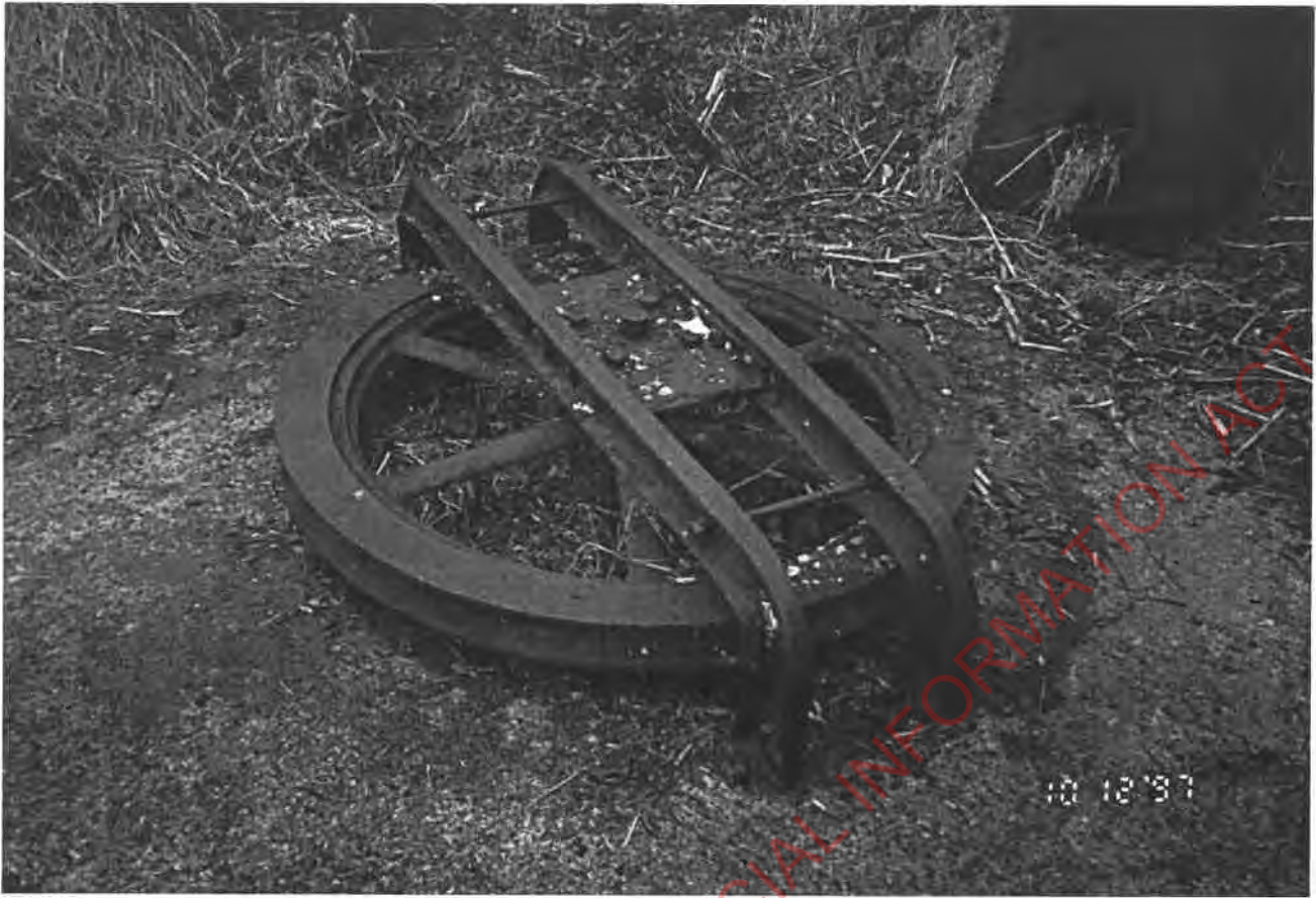
Figure 21: The incline wheel set into the rear of the upper road on the line of the tramway
