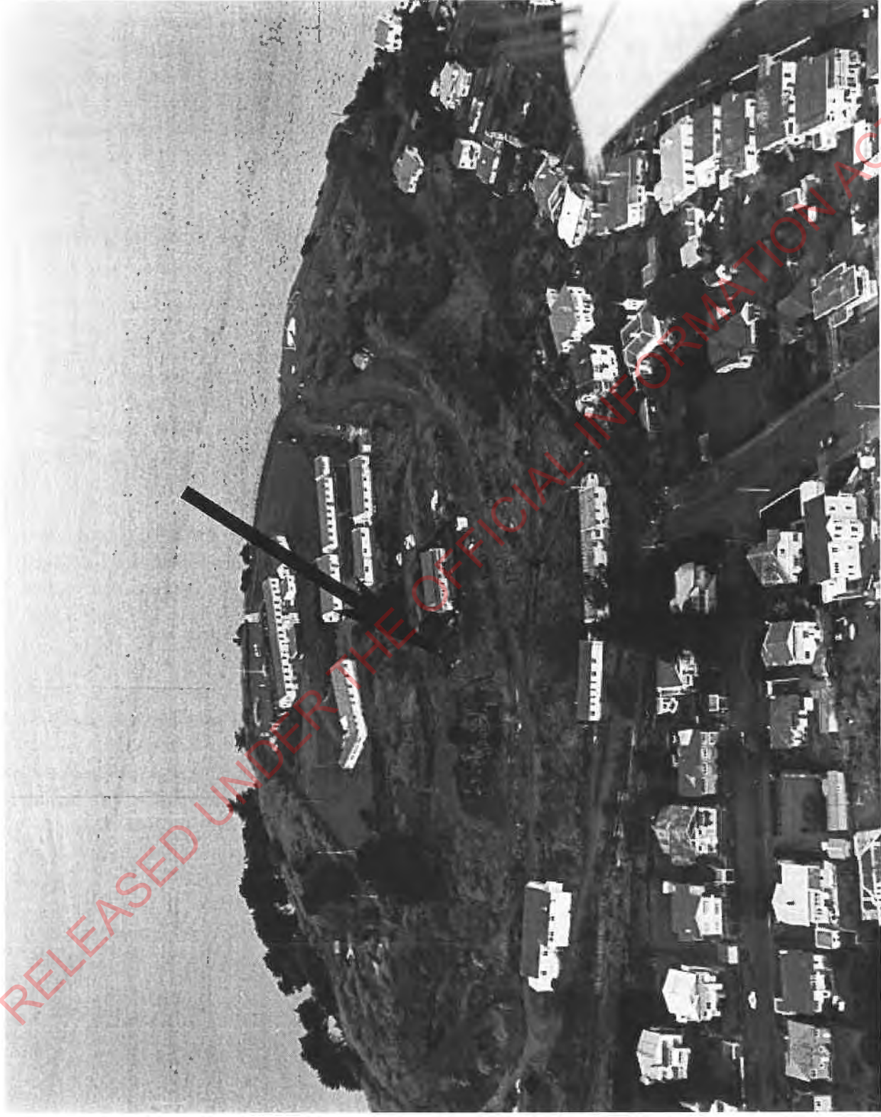
Figure 19: The structure on the western slope.
