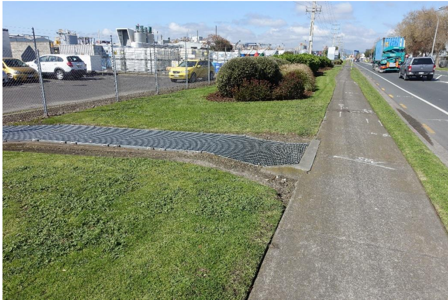
Figure 16: Drainage structure outside 2 Triton Avenue
