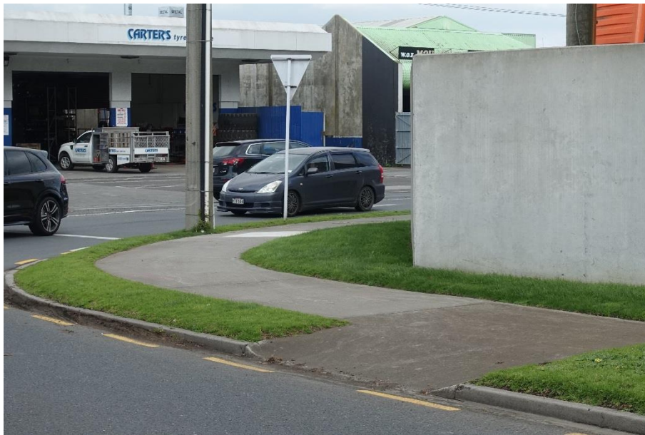
Figure 17: Poor intervisibility from the western crossing point at Hull Road roundabout
