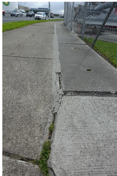
Figure 13: Broken service cover seal (Hewletts / Totara n-w quadrant)
