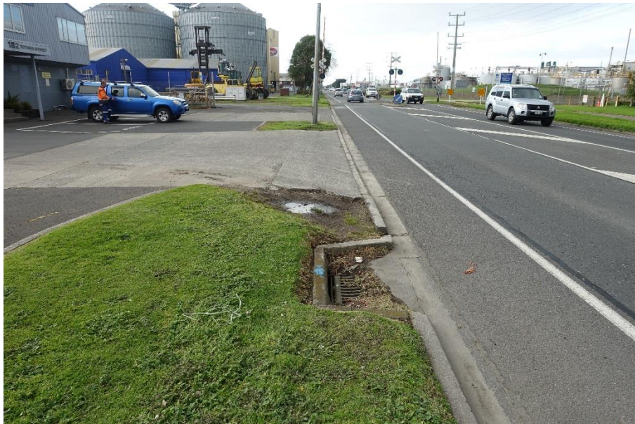
Figure 4: Chamfer created by truck overrun (driveway 9; Bulk Storage Terminals Ltd)
