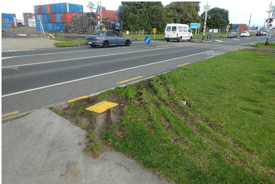
Figure 15: Splitter island geometrically constraining driveway 11
