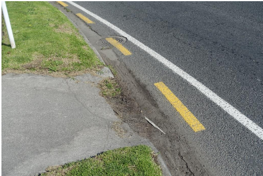
Figure 19: Mud accumulates at the pedestrian crossing point outside Carters Tyre Service
