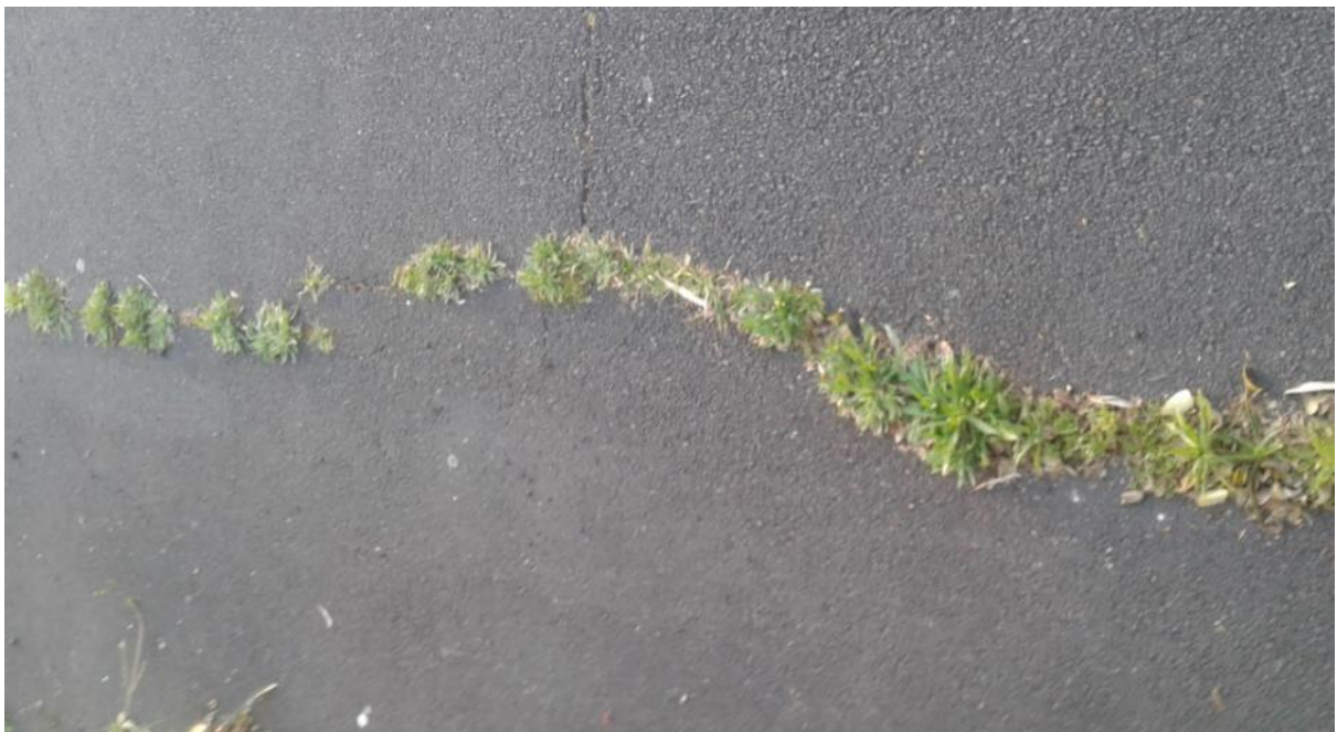
Figure 4 Weeds growing through a crack in the tarseal
