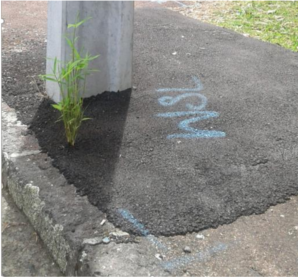
Figure 3 Bamboo growing through tarseal
