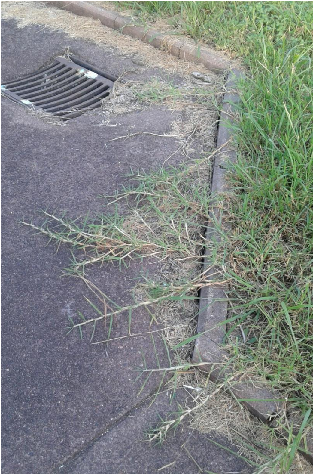
Figure 1 Kikuyu grass growing over the pavement
