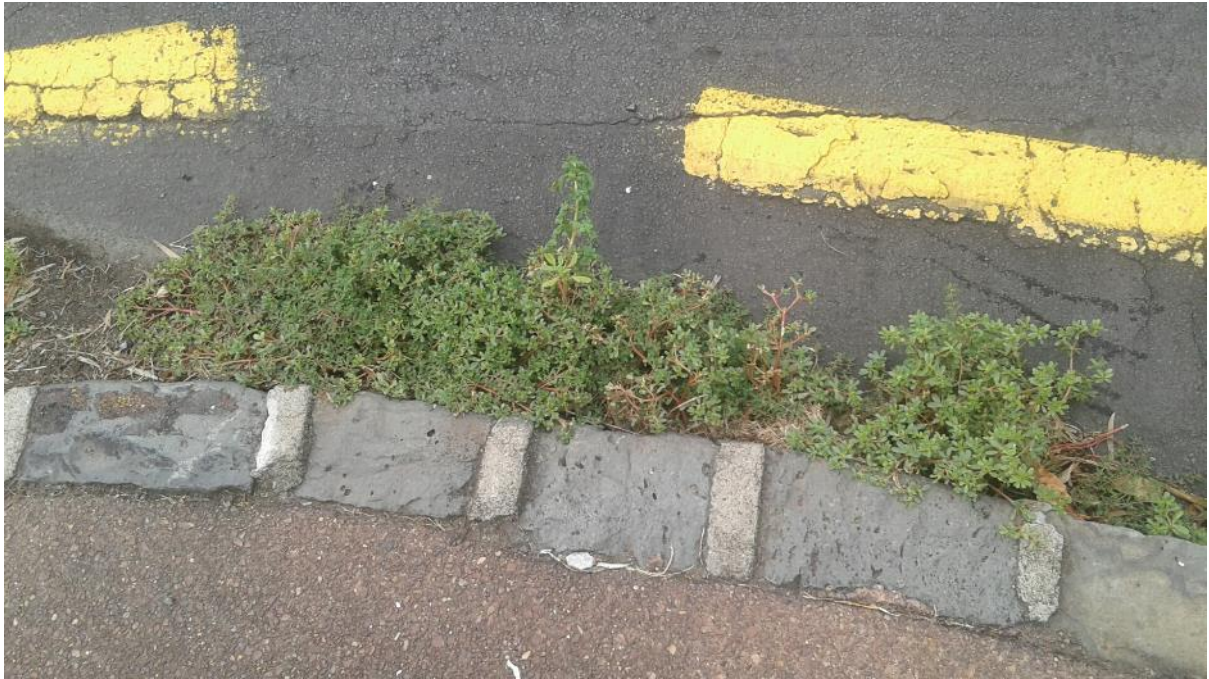
Figure 1 Weeds in the kerb and channel
