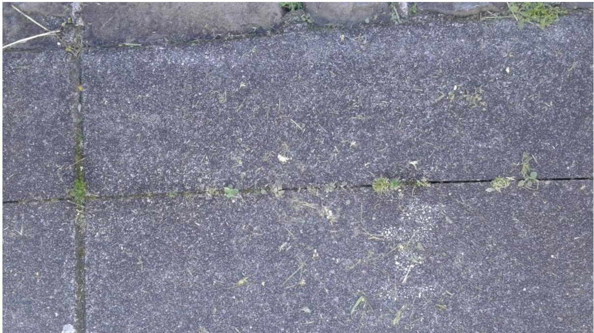
Figure 2 Vegetation growing in concrete expansion joints
