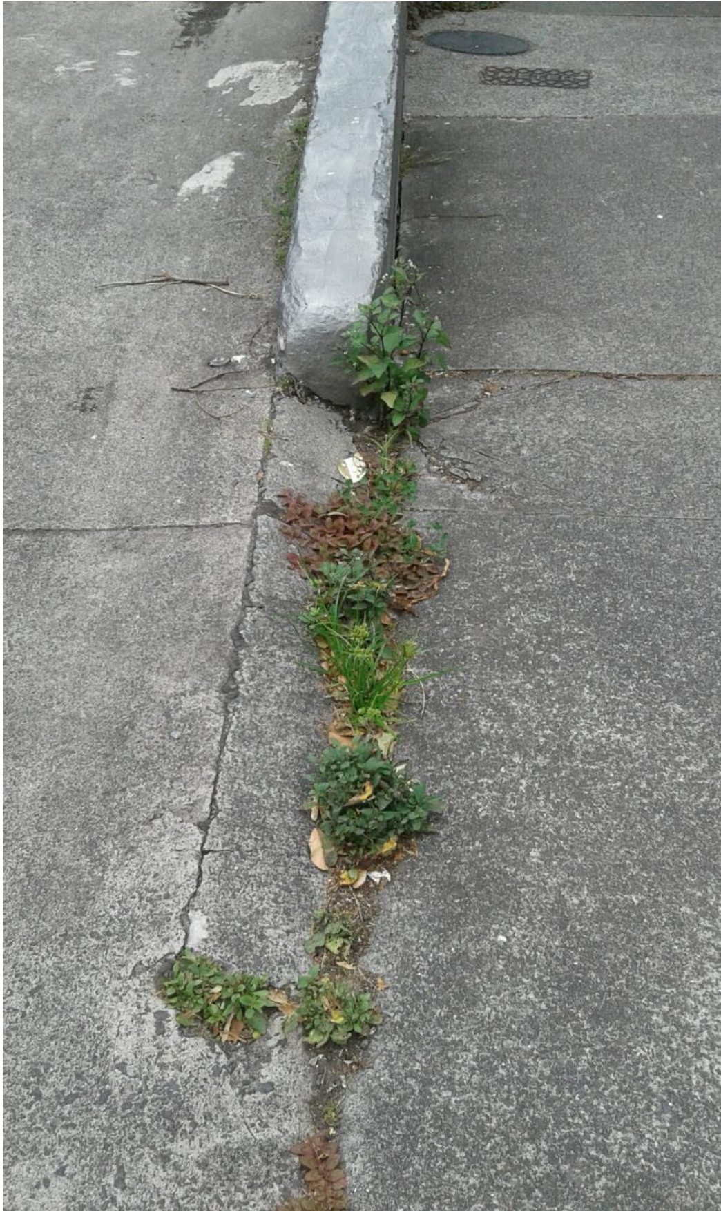
Figure 2 Weeds in the kerb and channel
