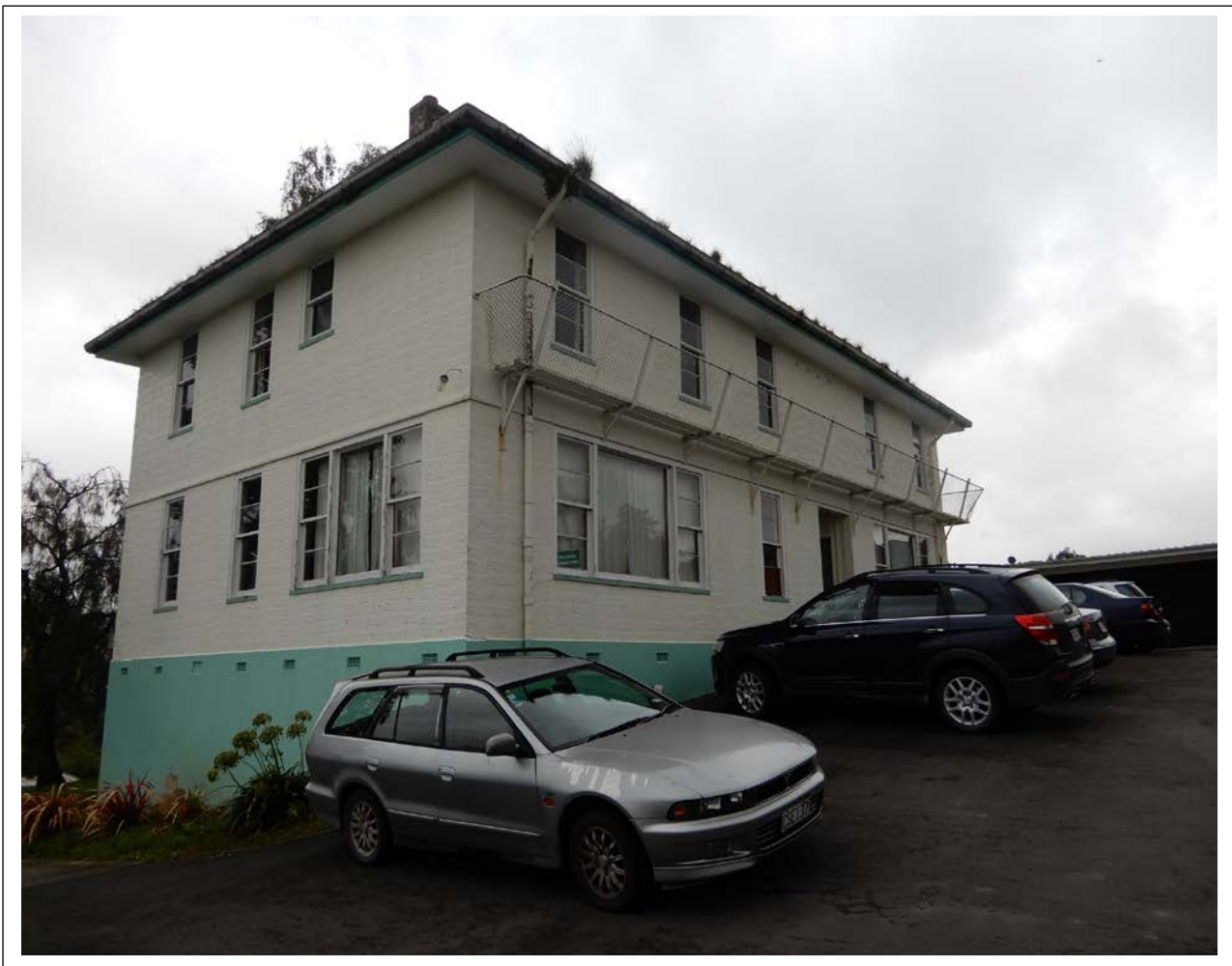
STAFF QUARTERS, TAIHAPE HOSPITAL.
