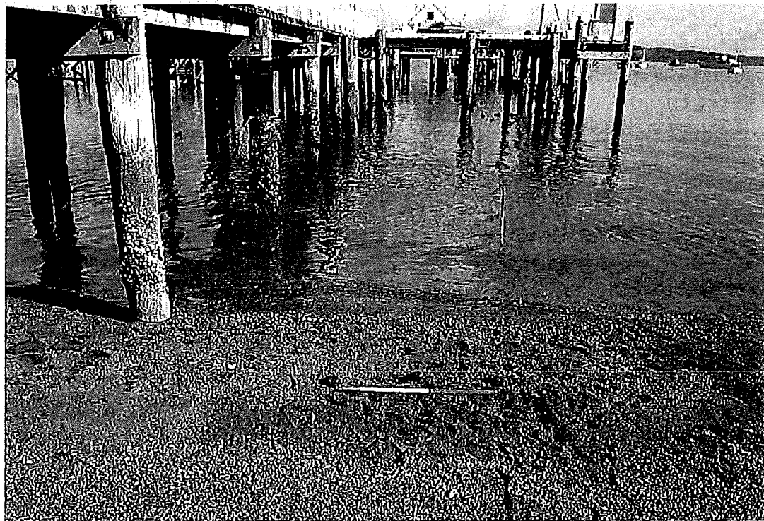
Plate 14: The small timber piles located at the low tide mark to the north of the current Russell wharf
