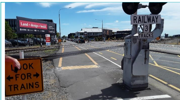
Figure 6: Tactile indicators installed behind the flashing lights and bells assembly on the eastern crossing
