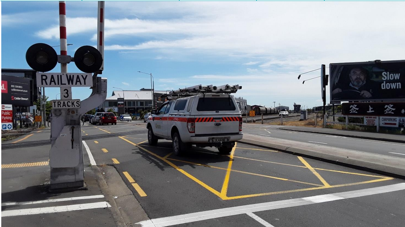
Figure 4: Traffic queues stacked across the multiple tracks within the rail corridor at the Lincoln Road level crossing
