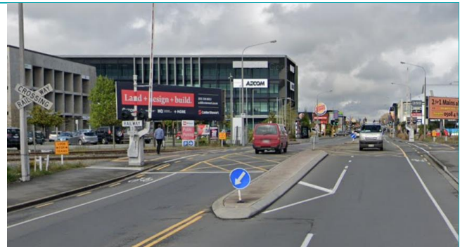
Figure 13: Vertical rise north of the rail corridor makes it difficult for drivers to judge whether there is enough space to clear the rail corridor when queues develop
