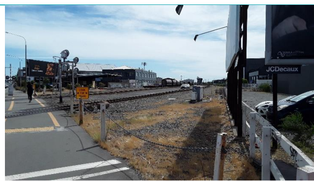
Figure 9: Pedestrian sight line from the western pedestrian crossing looking down track (west) is limited by the curve in the rail track
