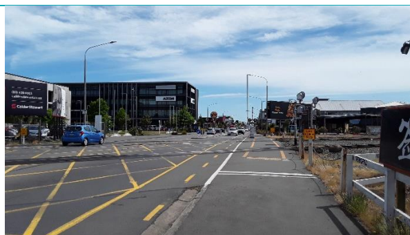
Figure 7: Western pedestrian crossing with passive warning control layout shown. There is no adjacent flashing lights and bells assembly on this approach
