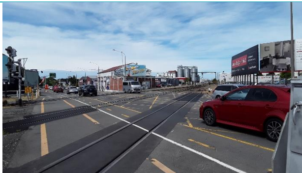
Figure 12: Queues forming at the Lincoln Road – Moorhouse Avenue signalised intersection stacking across multiple tracks at the Lincoln Road level crossing
