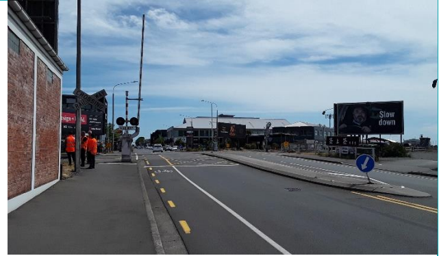
Figure 11: Southbound approach surface in good condition
