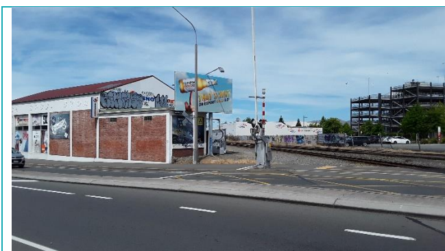
Figure 8: Pedestrian sight line from the western pedestrian crossing looking up track (east) severely restricted by property
