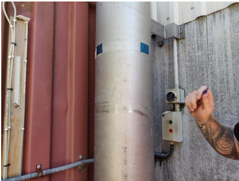
The blue tags are where emissions monitoring is conducted. The flow level is shown on the slide ruler.
