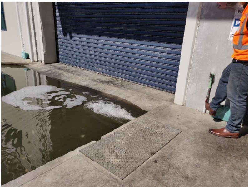
A demonstration of the truck wheel wash. The disinfectant is MPI-approved and contains iodine which stains the water red over time. Water collects in the depression before it drains away. Sometimes it may creep onto the concrete pad.
