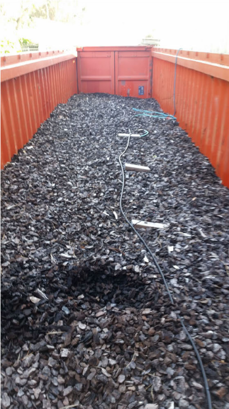
Figure 1 Interwaste biofilter surface
