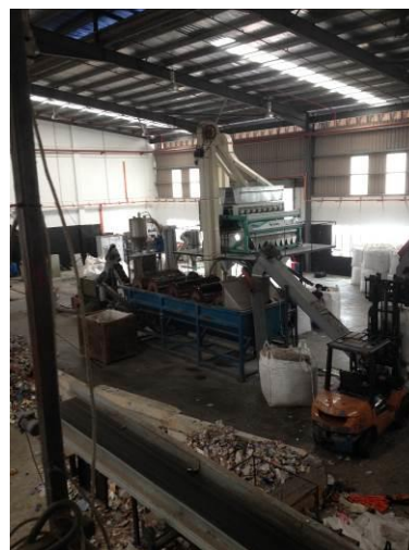
Automated sorting plant showing one of the optical sorting units.
