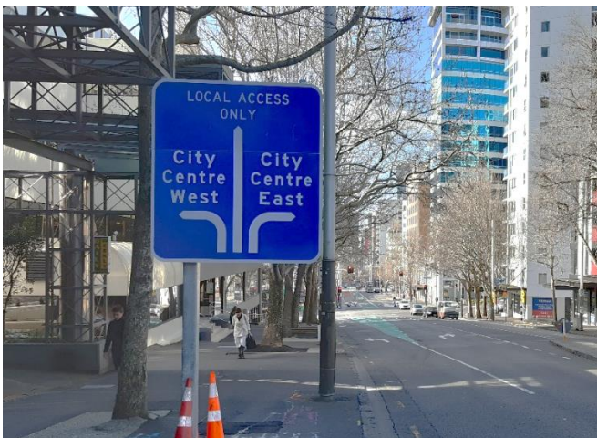
Figure 5: Advance direction stack sign installed between Karangahape Rd and Mayoral Drive (image provided by AT)
